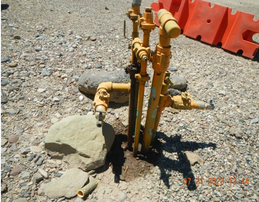
At group of unused flowlines north of the tank battery, a line with a leaky valve was saturated with condensate and stained ground.
