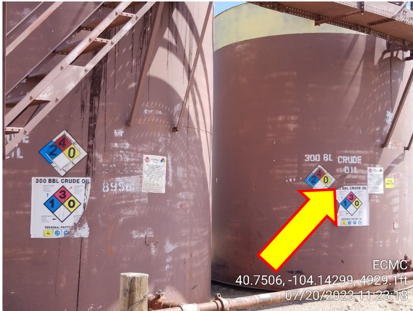
Photo 5 – East Tank – Capacity Label no longer visible
