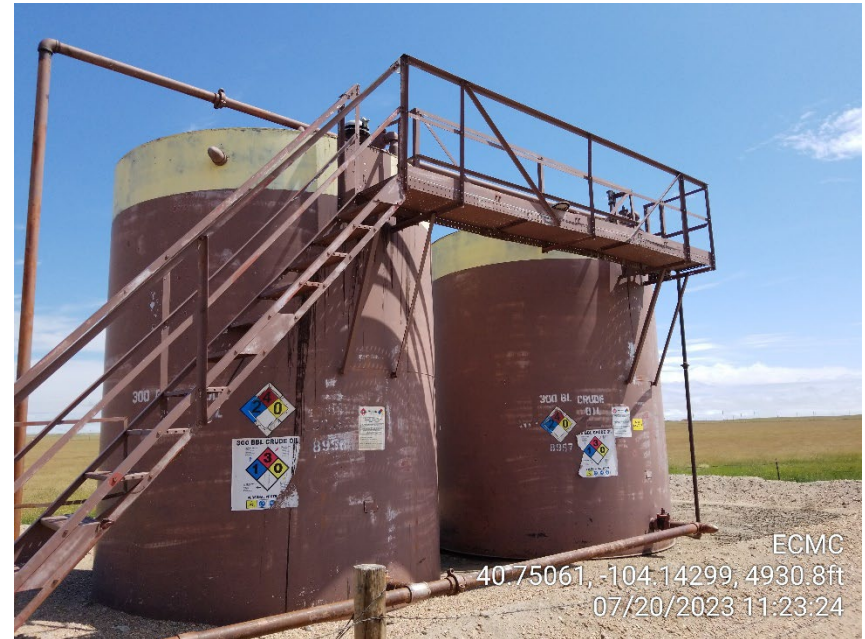
Photo 6 – Tank Battery
