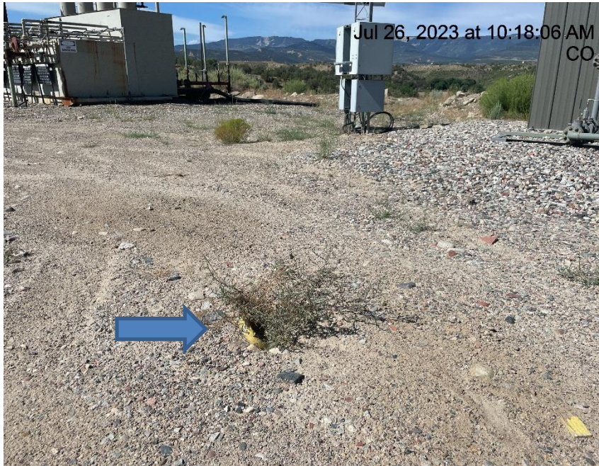
Photo # 3772 Same unmarked deadman from a different angle
