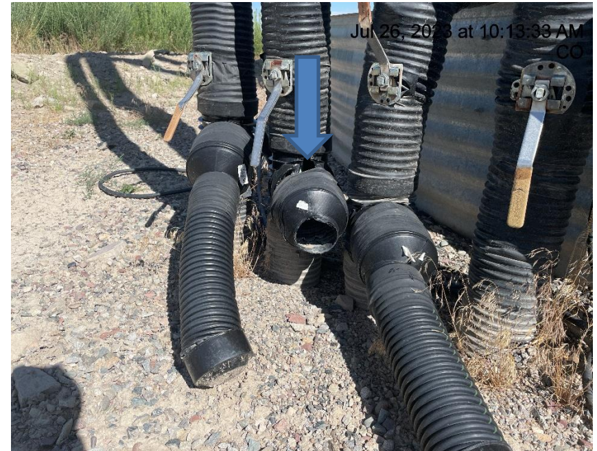
Photo # 3762 Flowline heating insulation open ended
