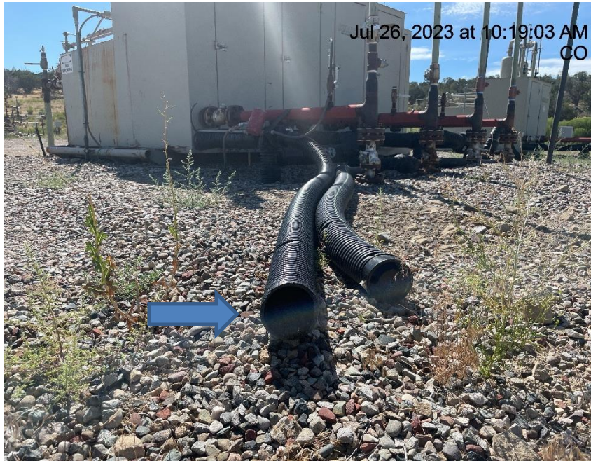
Photo # 3774 Flowline heating insulation open ended
