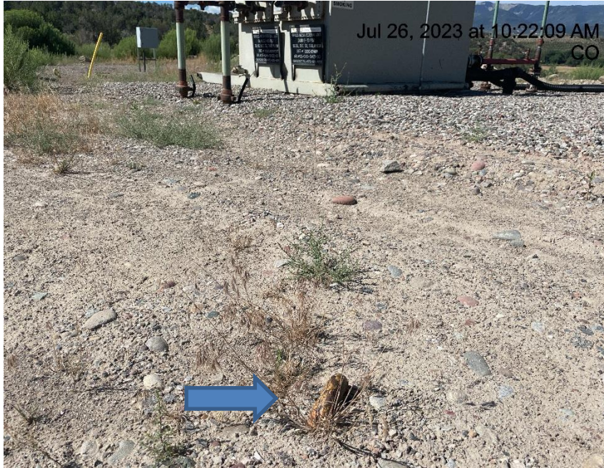
Photo # 3776 Same unmarked deadman from a different angle
