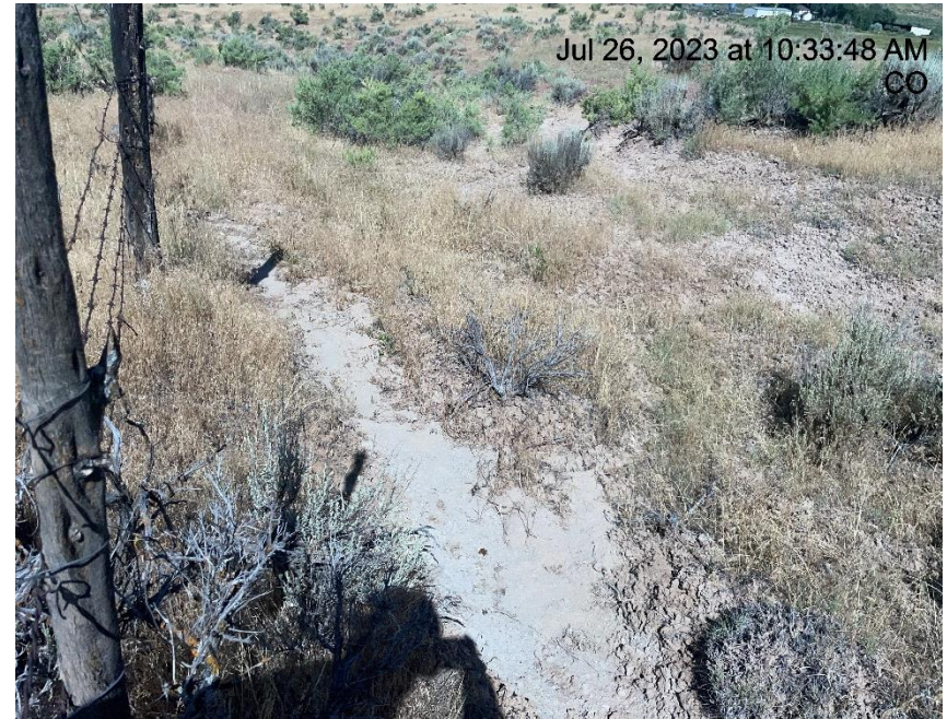
Photo # 3795 Failure to minimize erosion & transport of sediment/sediment choking off vegetation
