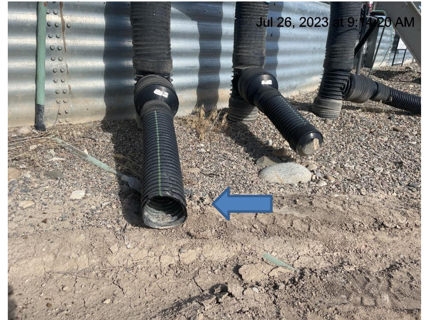
Photo # 3726 Flowline heating insulation open ended
