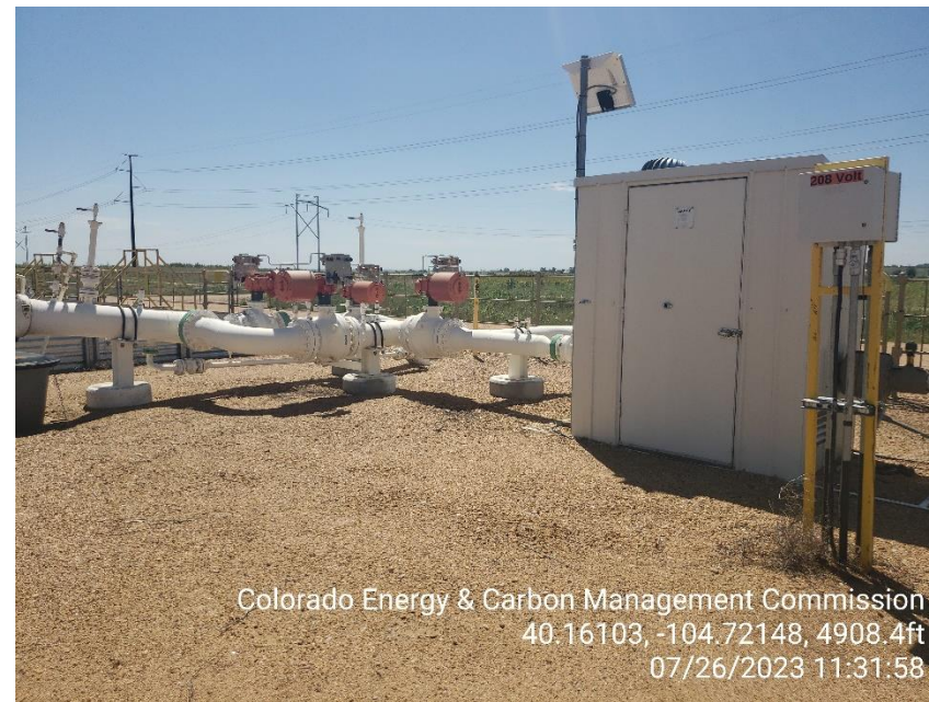
Photo 16 Gas Meter Run.
