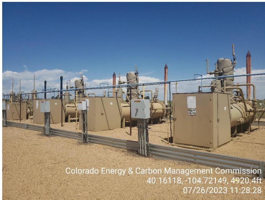
Photo 7 Horizontal Heated separators.
