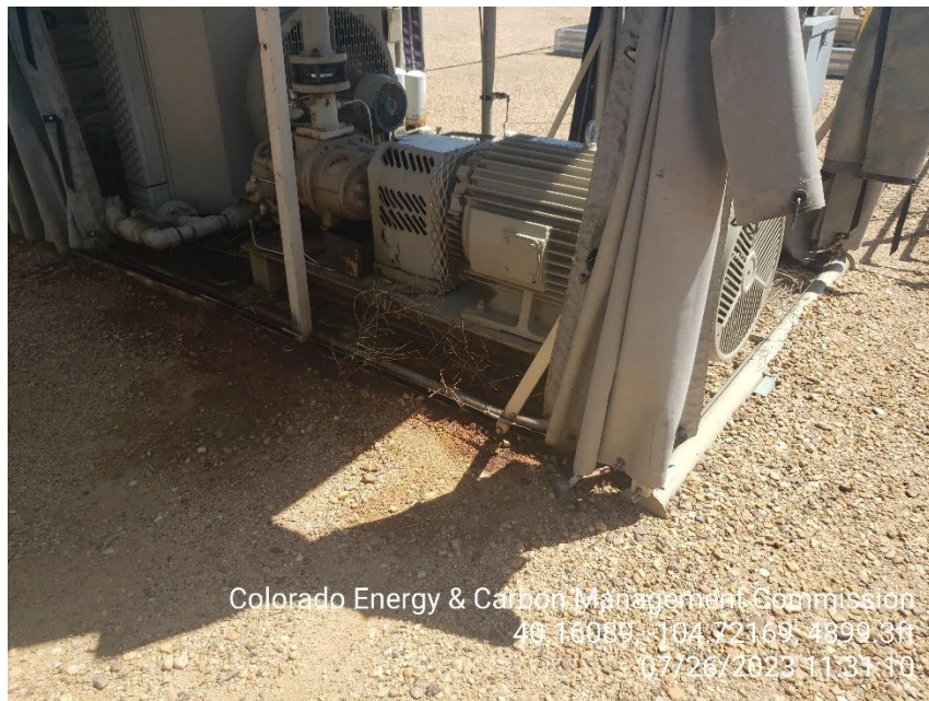
Photo 11 Stained soil around the east VRU.
