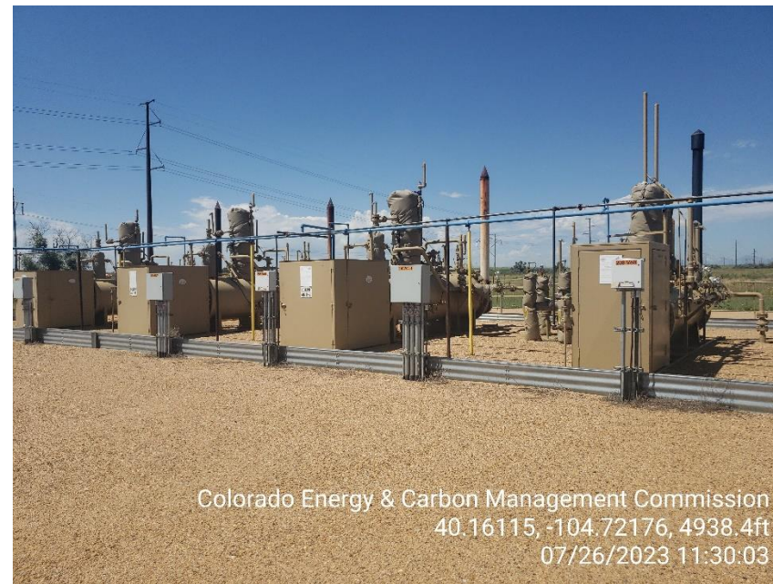
Photo 8 Horizontal Heated separators.
