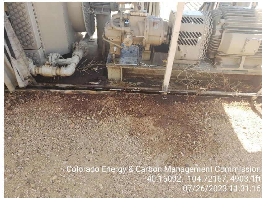
Photo 12 Stained soil around the east VRU.
