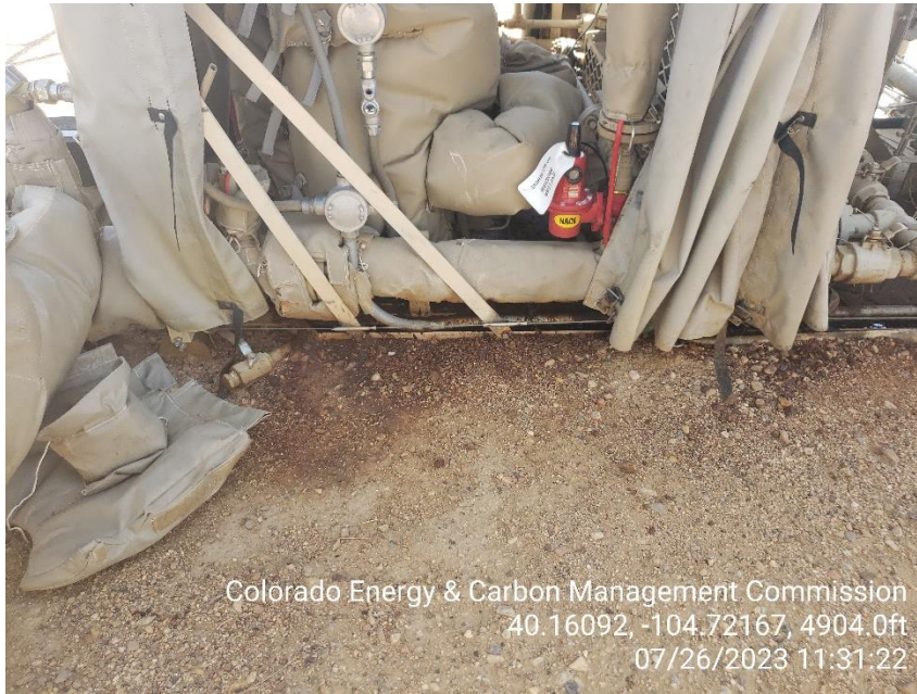
Photo 13 Stained soil around the east VRU.
