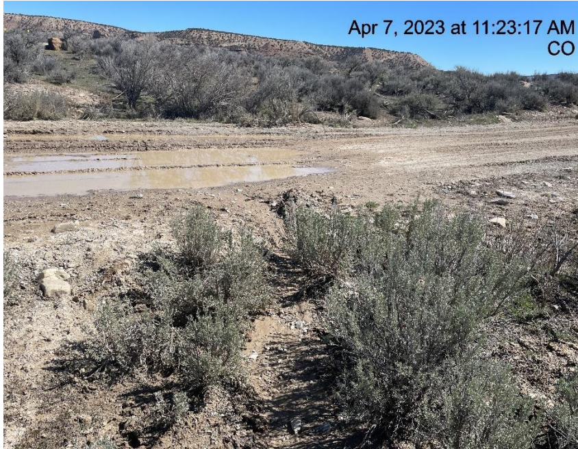
Photo # 4640 From Inspection 708900241 conducted on 04/07/2023 Erosion & transport of sediment off lease road/insufficient BMP's
