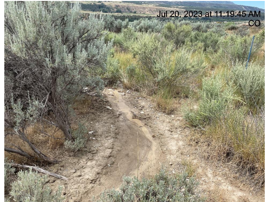
Photo # 3494 Erosion & transport of sediment off lease road/insufficient BMP's – sediment is being transported into a vegetated area & choking off vegetation.
