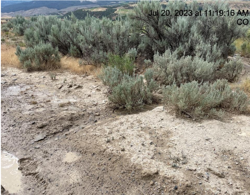
Photo # 3490 Erosion & transport of sediment off lease road/insufficient BMP's
