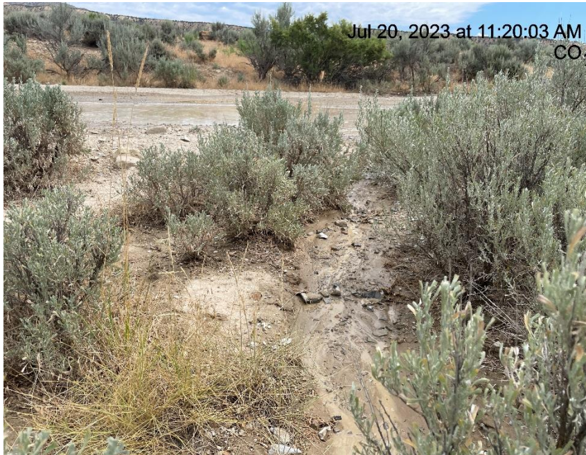
Photo # 3493 Erosion & transport of sediment off lease road/insufficient BMP's – sediment is being transported into a vegetated area & choking off vegetation.
