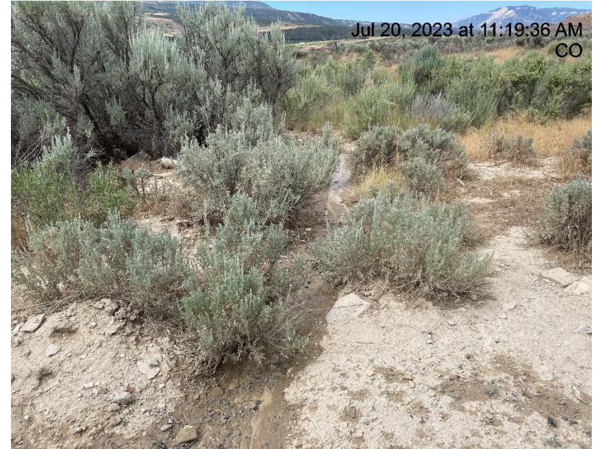
Photo # 3492 Erosion & transport of sediment off lease road/insufficient BMP's
