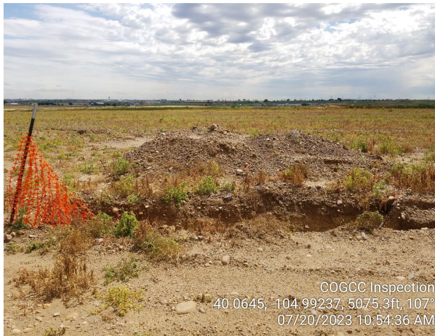
Photo 13 – Flowline excavation for Rem 26277. Fencing is down around open excavation. Soil stockpile has missing/inadequate BMPs.
