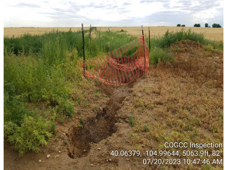
Photo 4 – Flowline excavation for Rem 26277. Fencing is down around open excavation. Soil stockpile has missing/inadequate BMPs. Weeds on access road for API 05-123-09913.
