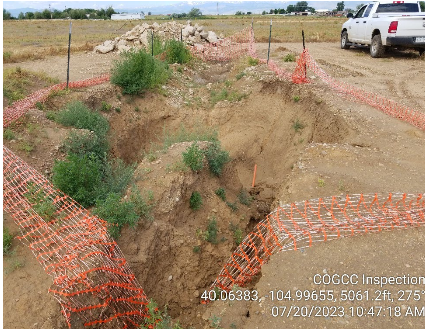
Photo 15 – Wellhead (API 05-123-09913) excavation for Rem 26277. Fencing is down around open excavation. Trash and debris (concrete, rebar, etc.) piled near open excavation.
