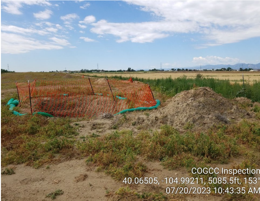
Photo 1 – Spill ID 481679 excavation. Fencing is falling down around open excavation. Soil stored on location with inadequate BMPs.
