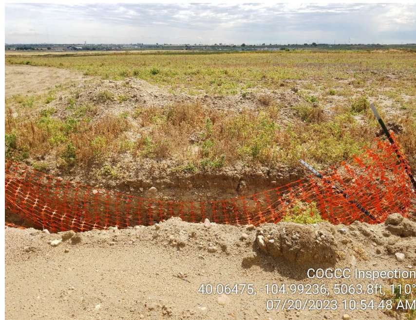
Photo 14 – Flowline excavation for Rem 26277. Fencing is down around open excavation.
