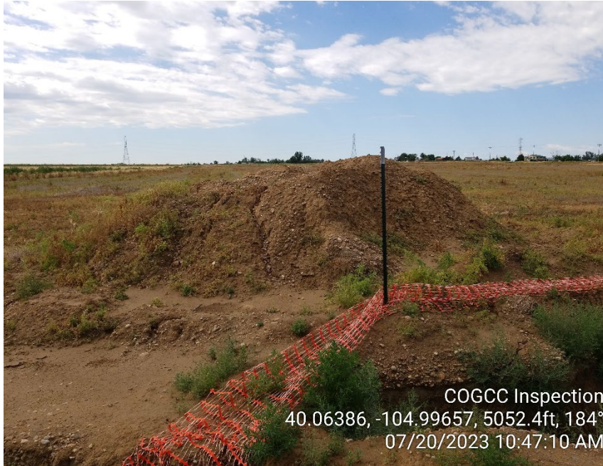
Photo 17 – Soils pile with no BMPs present next to open wellhead excavation.
