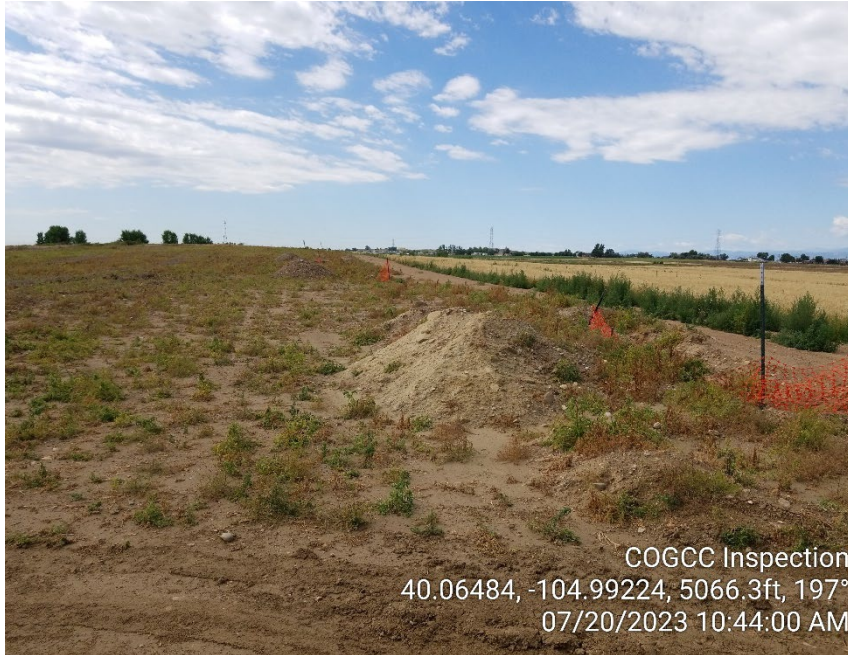
Photo 3 – Flowline excavation for Rem 26277. Fencing is down around open excavation. Soil stockpile has missing/inadequate BMPs.
