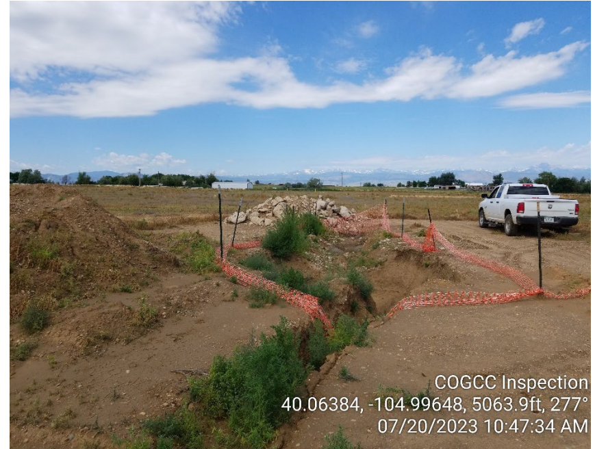
Photo 16 – Wellhead (API 05-123-09913) excavation for Rem 26277. Fencing is down around open excavation. Trash and debris (concrete, rebar, etc.) piled near open excavation. Weeds growing in open excavation. Soils pile with no BMPs present next to open excavation.
