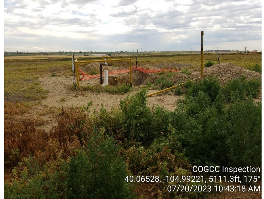
Photo 2 – Flowline excavation for Rem 26277. Fencing is down around open excavation. Soil stockpile has missing/inadequate BMPs.
