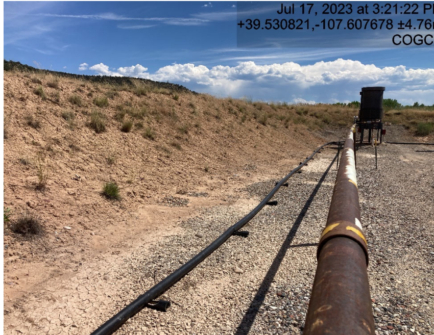
Cut slope shows signs of lack of stabilization and erosion
