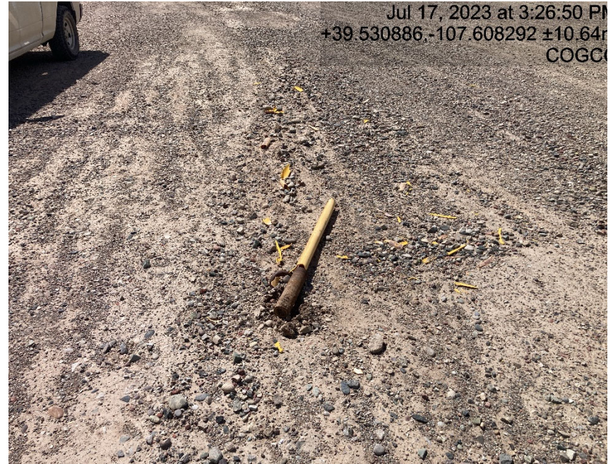
Dead man not marked properly and random debris
