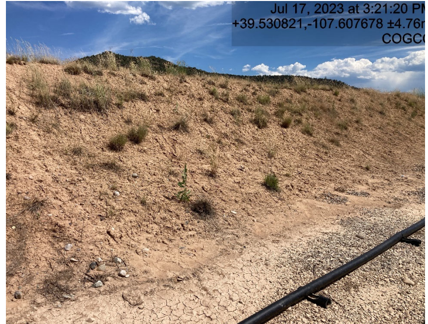
Cut slope shows signs of lack of stabilization and erosion
