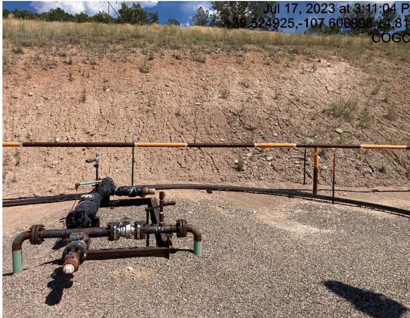
Lack of stabilization and rill erosion
