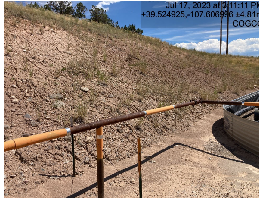
Lack of stabilization and rill erosion
