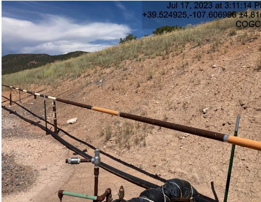
Lack of stabilization and rill erosion
