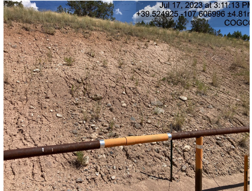
Lack of stabilization and rill erosion
