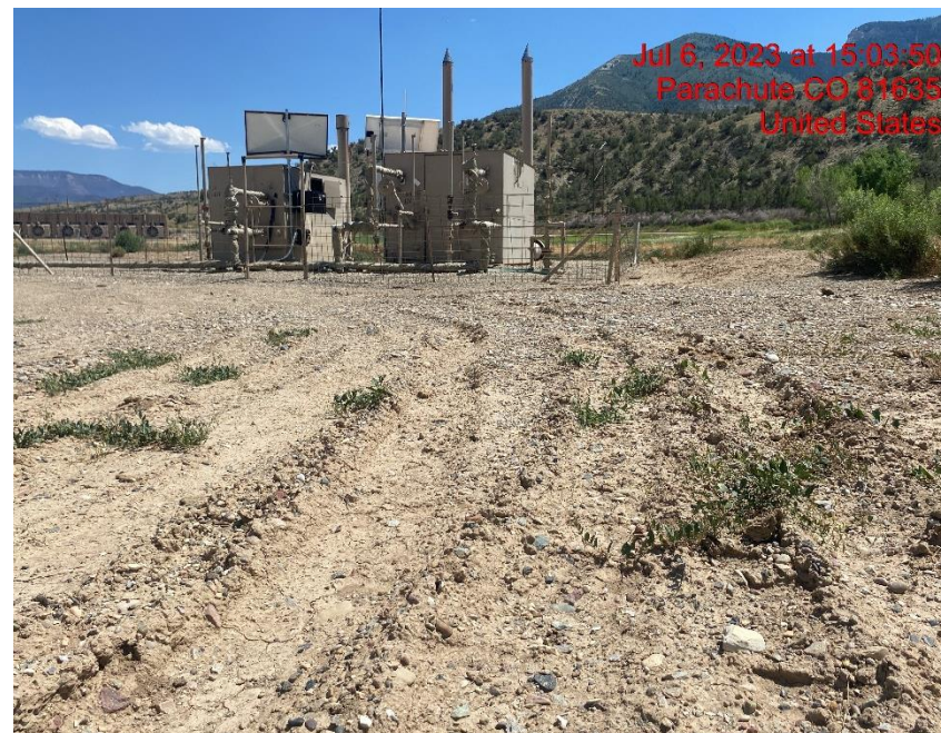
Lack of Stabilization – Photo #05044
