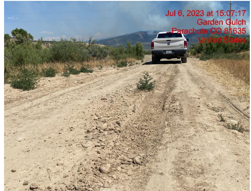
Lack of Stabilization on Access Road – Photo #05049
