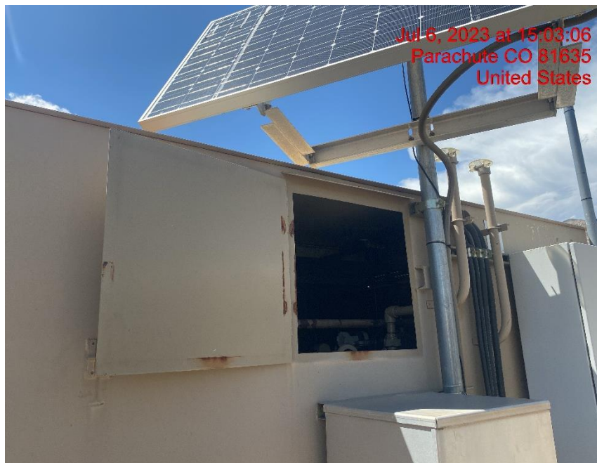
Unsecured Hatch on Separator – Photo #05043
