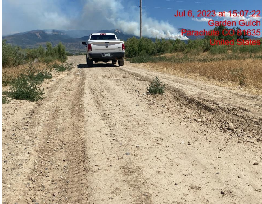
Lack of Stabilization on Access Road – Photo #05050
