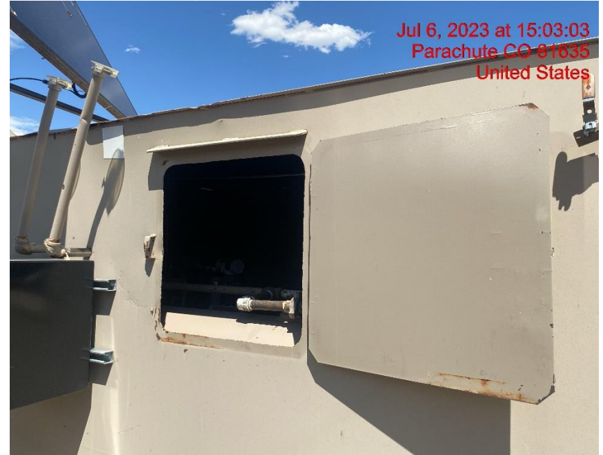
Unsecured Hatch on Separator – Photo #05042
