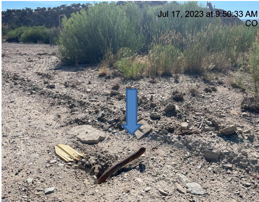
Photo # 3154 Debris/Hazard - broken deadman/anchor sticking up out of the ground
