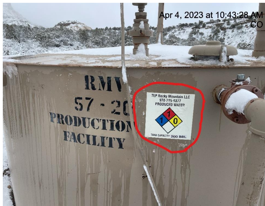
Photo # 4230 From Inspection 708900232 conducted on 04/04/2023 Tank label has incorrect information
