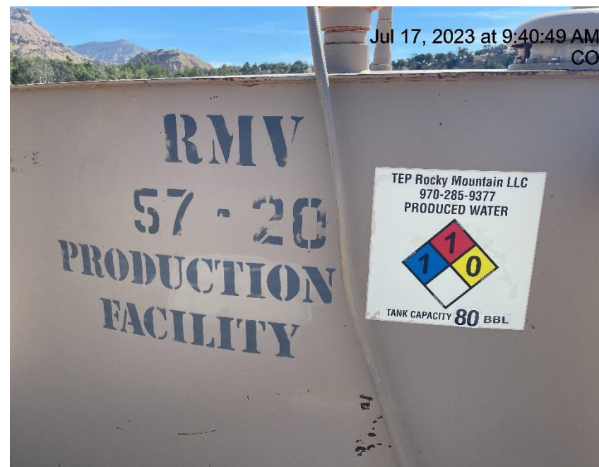
Photo # 3145 Tank label has incorrect information/capacity incorrect
