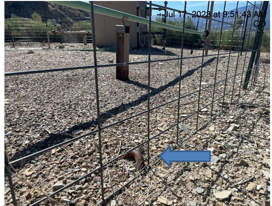
Photo # 3157 Same unmarked deadman/anchor from a different angle
