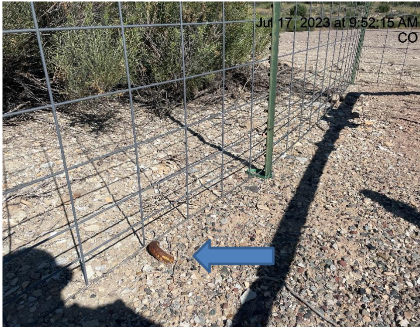
Photo # 3158 Unmarked deadman/anchor
