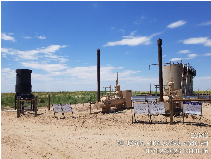
Photo 1 – Separators and ECD
