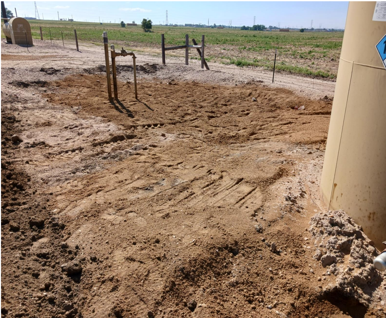
Figure #2 Stained soil removed; marked riser;
