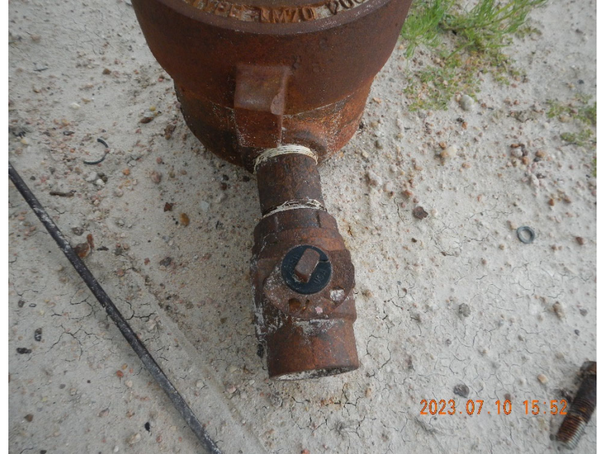
8. Surface casing valve open to atmosphere.
