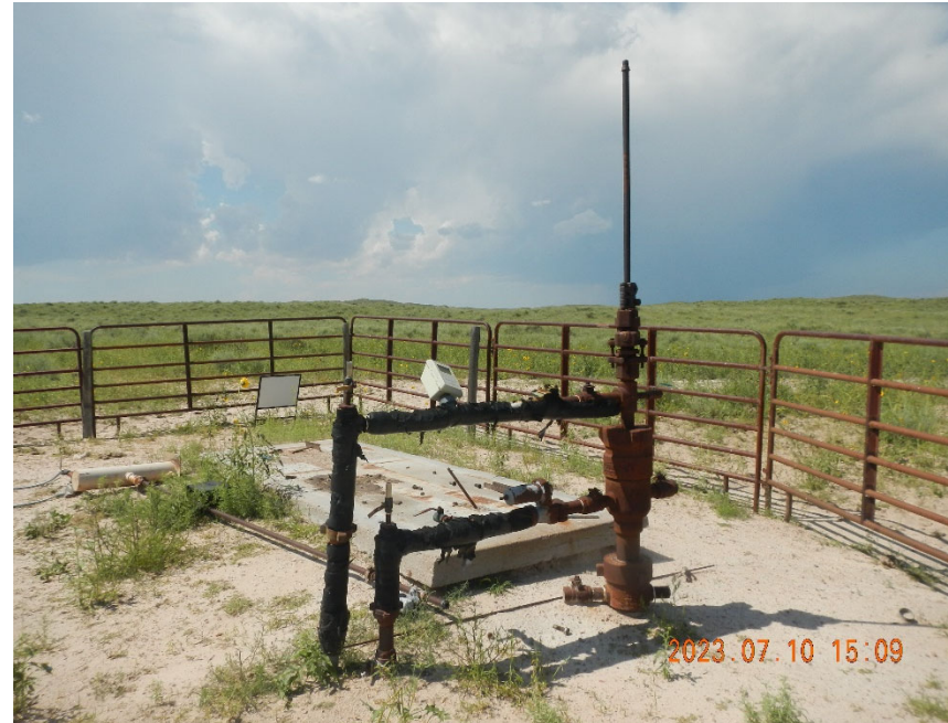
2. View of wellhead with polish rod visible.
