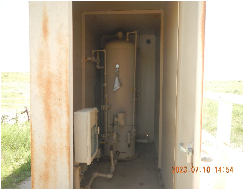
5. View of Gas Meter Run and Vertical Separator inside shed.
