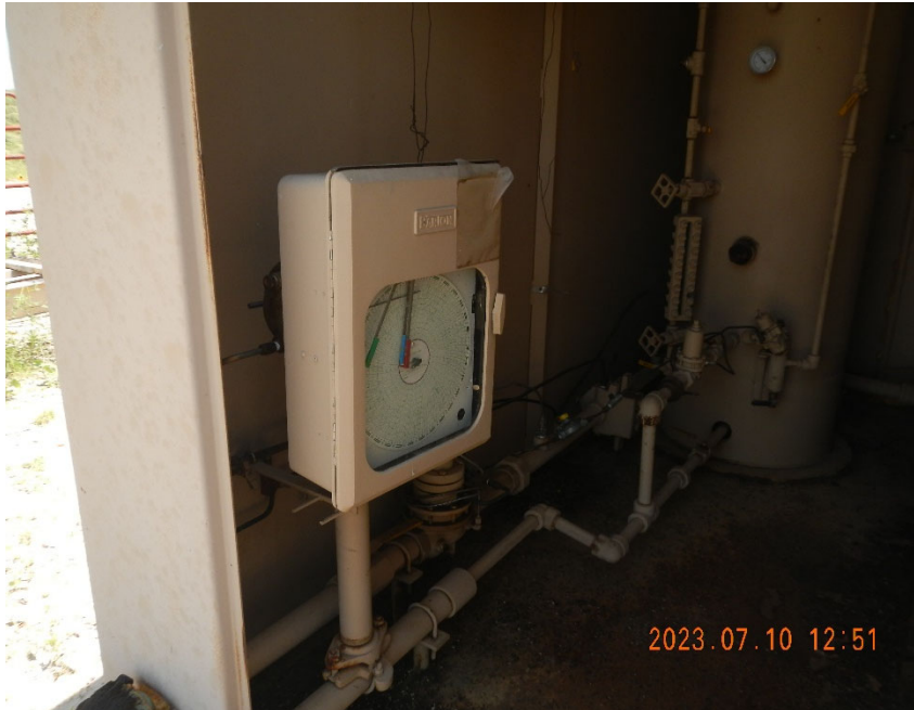
5. Meter/Separator building with door open and Gas Meter Run visible.
