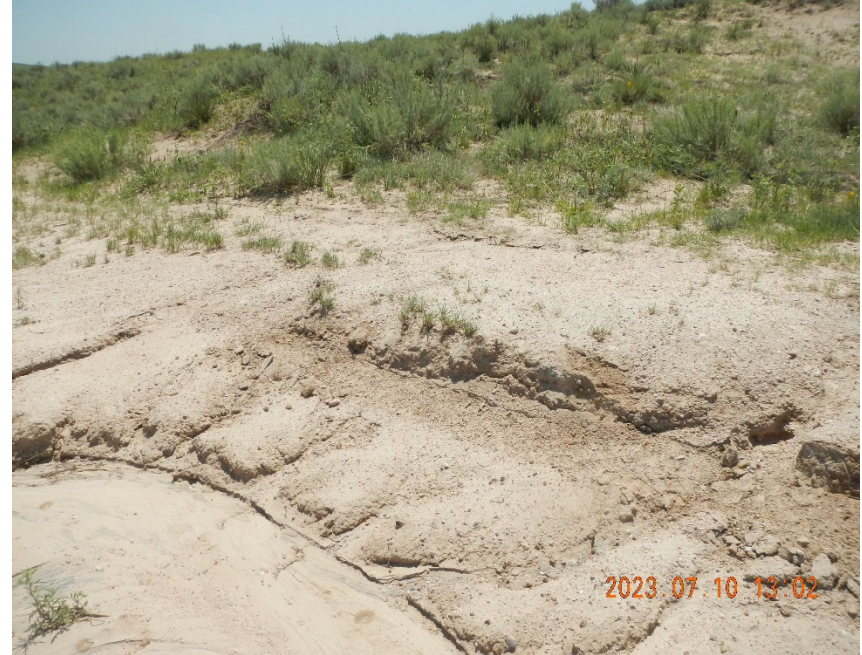
10. View of area where access road has washed out and erosion channel turns in more E direction carrying sediment down the sloping grade.
