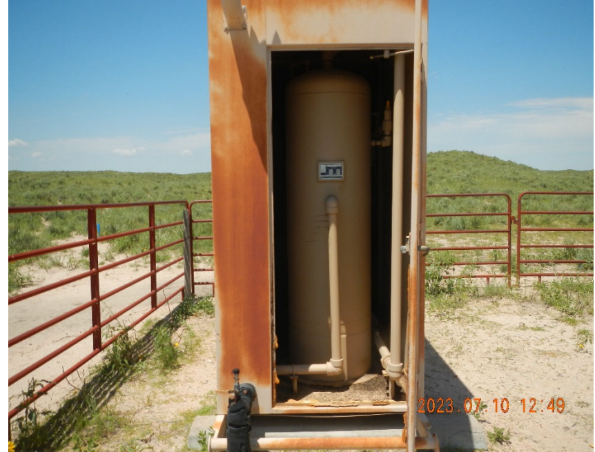
4. Meter/Separator building with door open and Vertical Separator visible.
