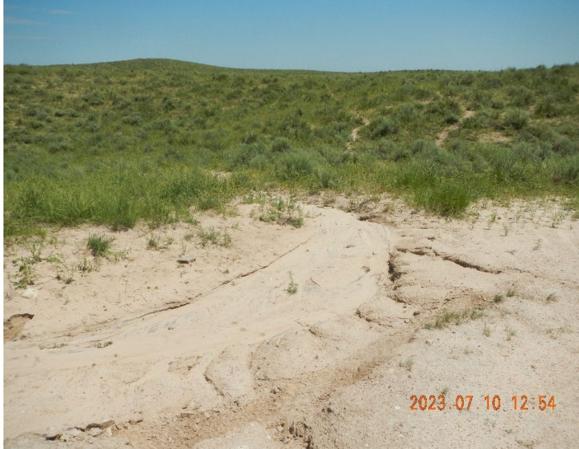
9. Closer view of erosion channel looking from location entry area to the SE down access road.
