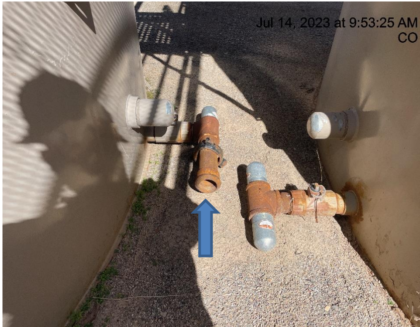
Photo # 3036 Open ended load line
