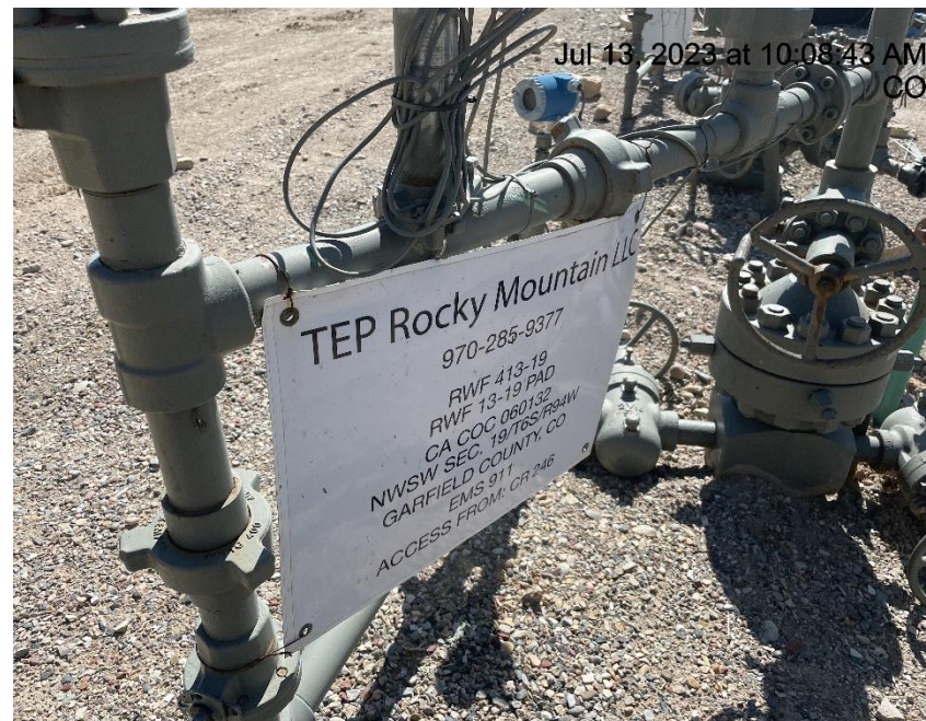
Photo # 2922 Wellhead sign missing API #
