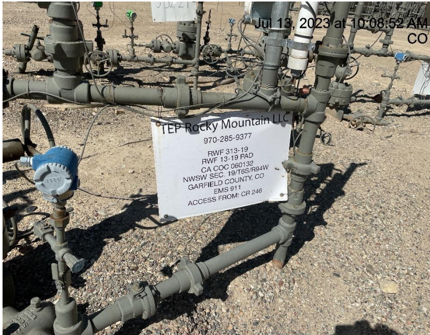
Photo # 2923 Wellhead sign missing API #
