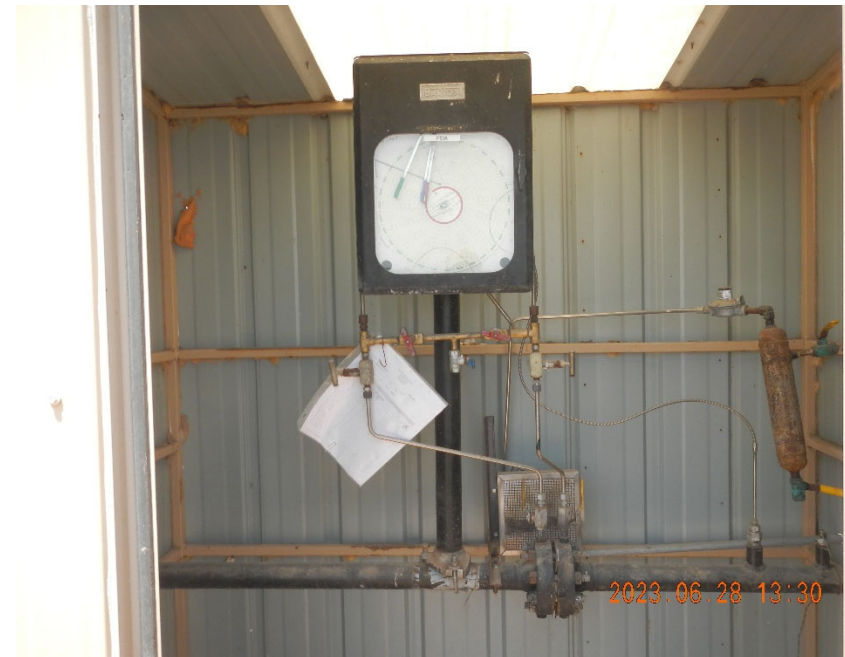
10. View of gas meter run inside meter shed.
