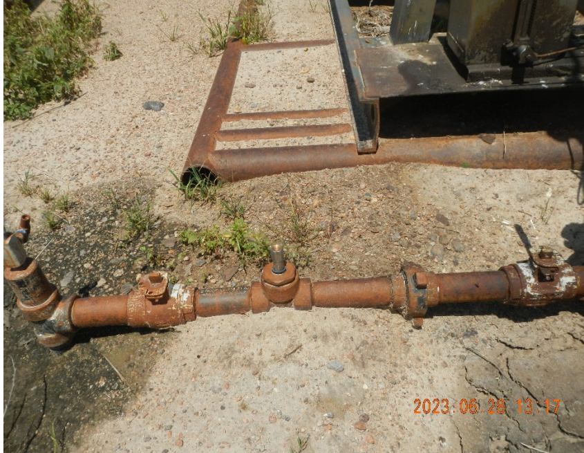
3. Casing flowline off west side of wellhead with visible soil staining.
