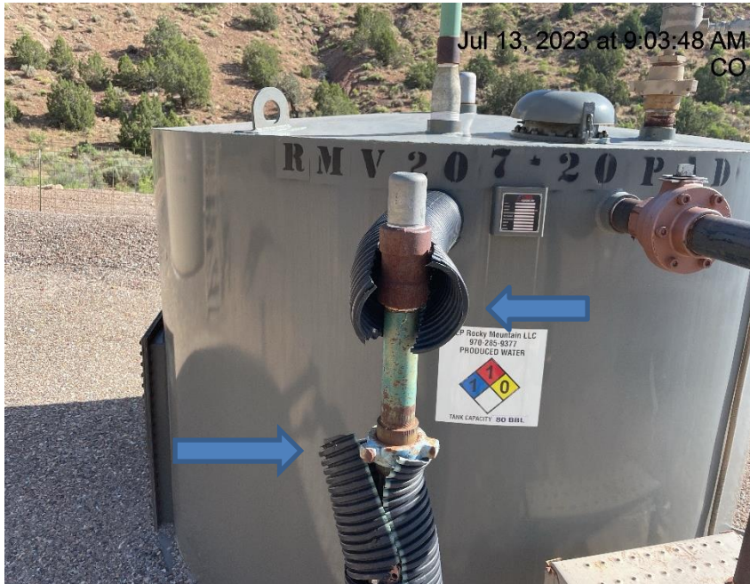
Photo # 2870 Flowline heating insulation open ended
