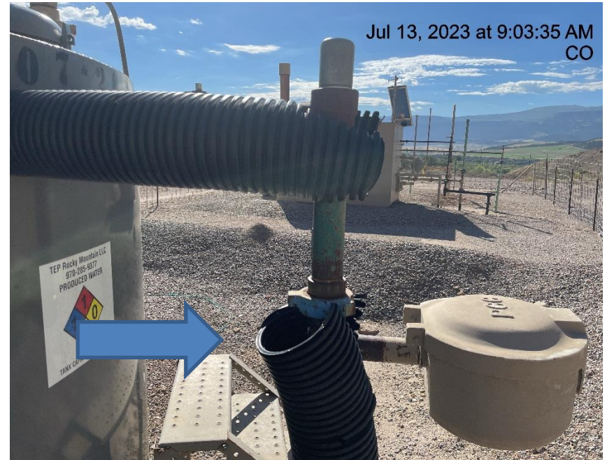
Photo # 2869 Flowline heating insulation open ended
