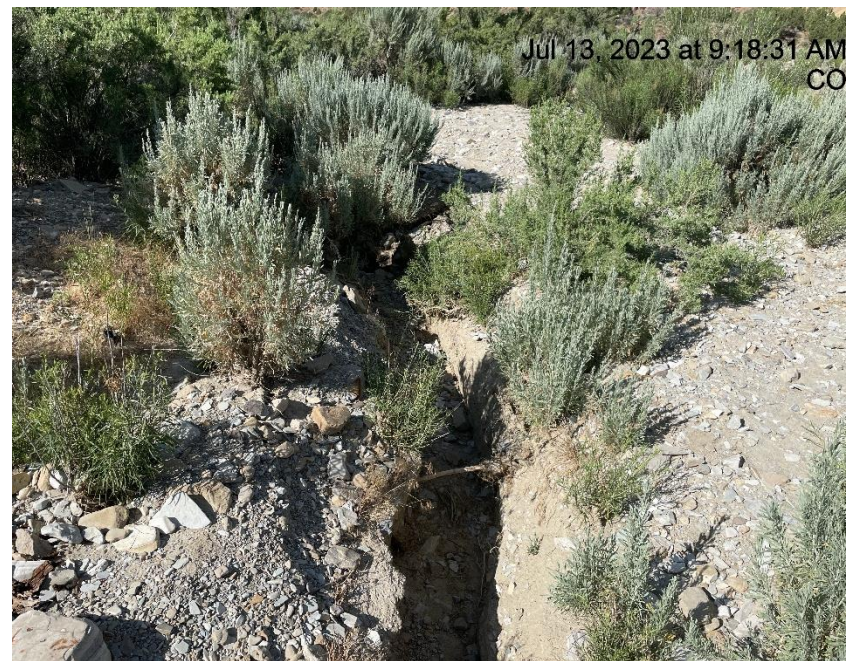
Photo # 2899 Erosion & transport of sediment (edge of lease road, approximately 1/10 th of a mile from location)
