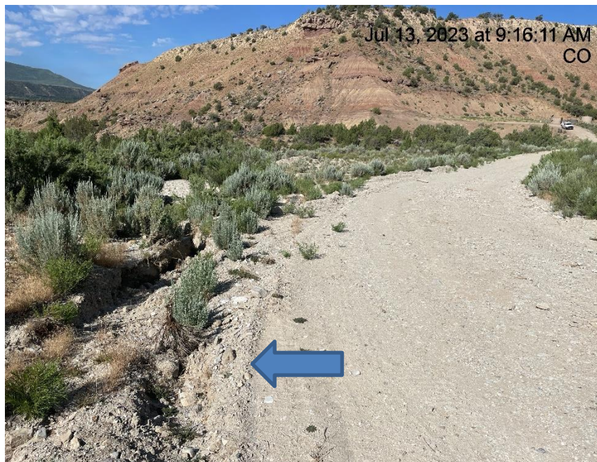
Photo # 2890 Erosion & transport of sediment (edge of lease road, approximately 1/10 th of a mile from location)
