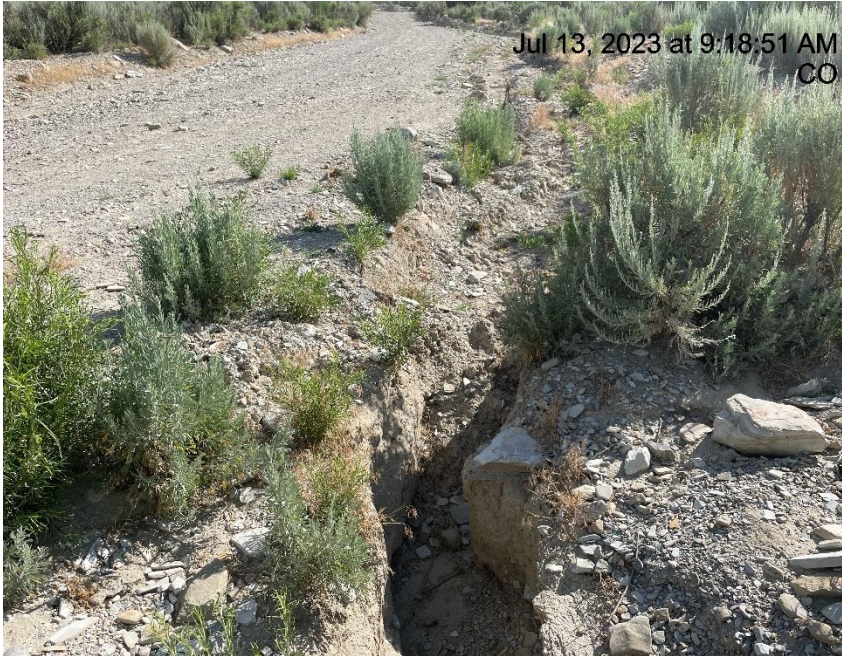
Photo # 2900 Erosion & transport of sediment (edge of lease road, approximately 1/10 th of a mile from location)
