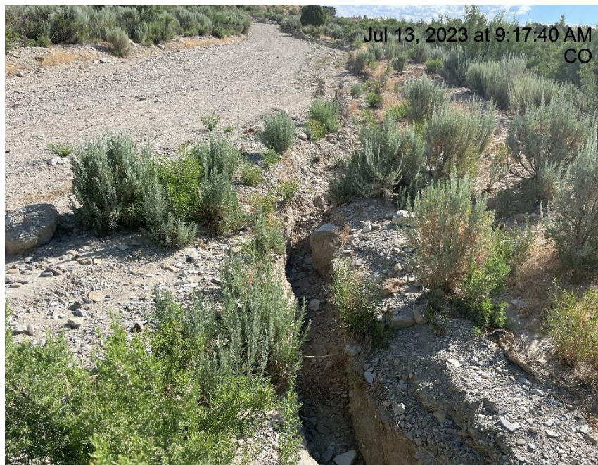
Photo # 2897 Erosion & transport of sediment (edge of lease road, approximately 1/10 th of a mile from location)
