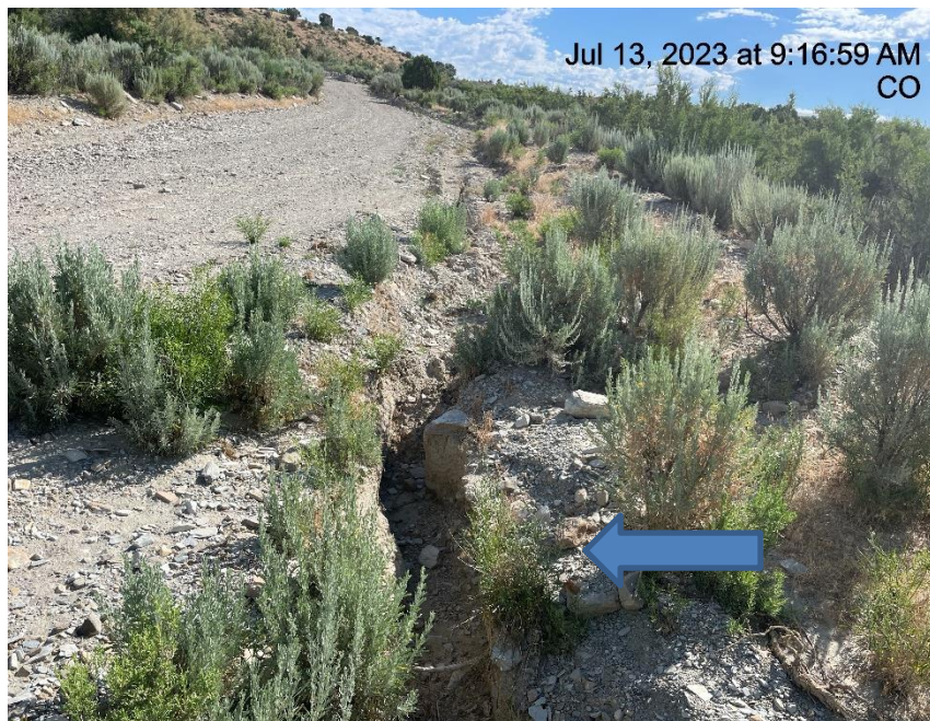
Photo # 2894 Erosion & transport of sediment (edge of lease road, approximately 1/10th of a mile from location)
