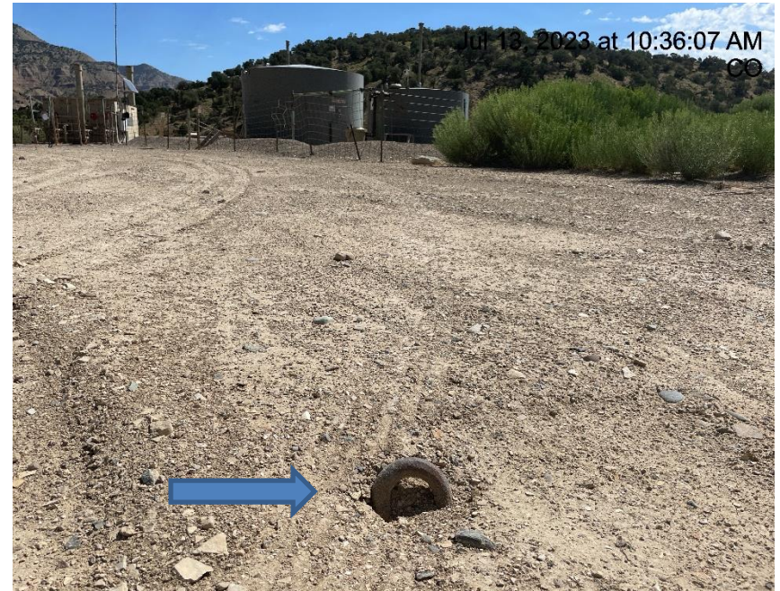
Photo # 2961 Same unmarked deadman from a different angle
