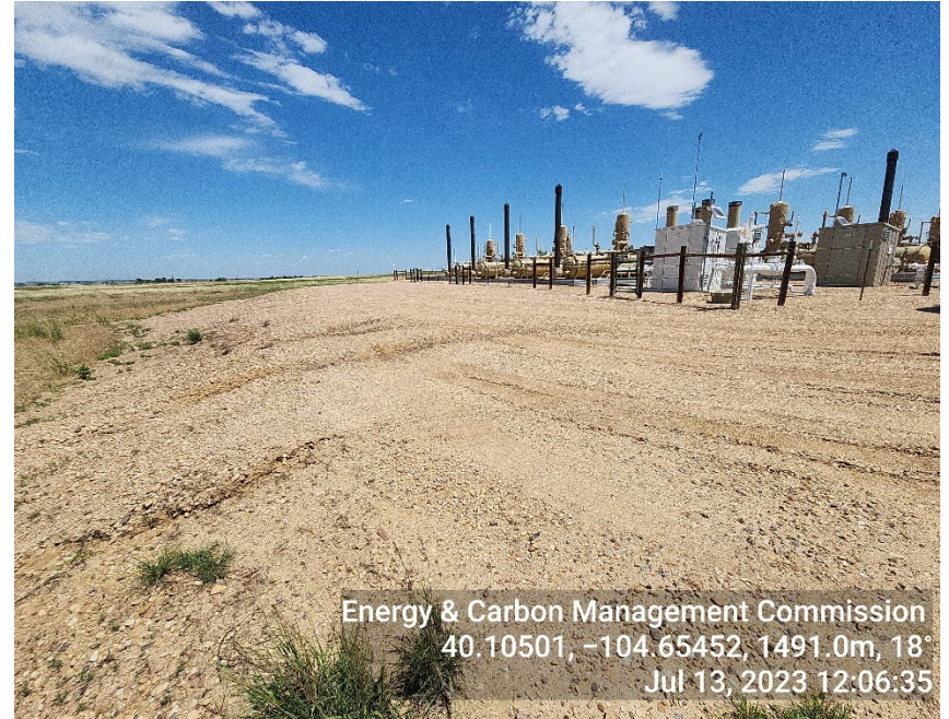
Photo 8: Erosion E of location (near gas meters)
