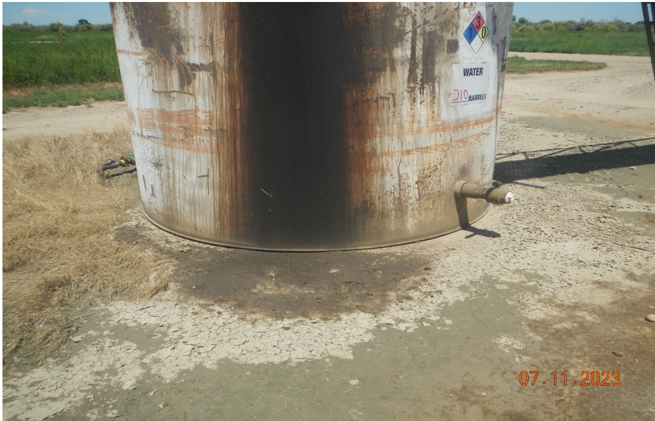
Photo 3. There is oil stained soils at the tank that need to be cleaned up.
