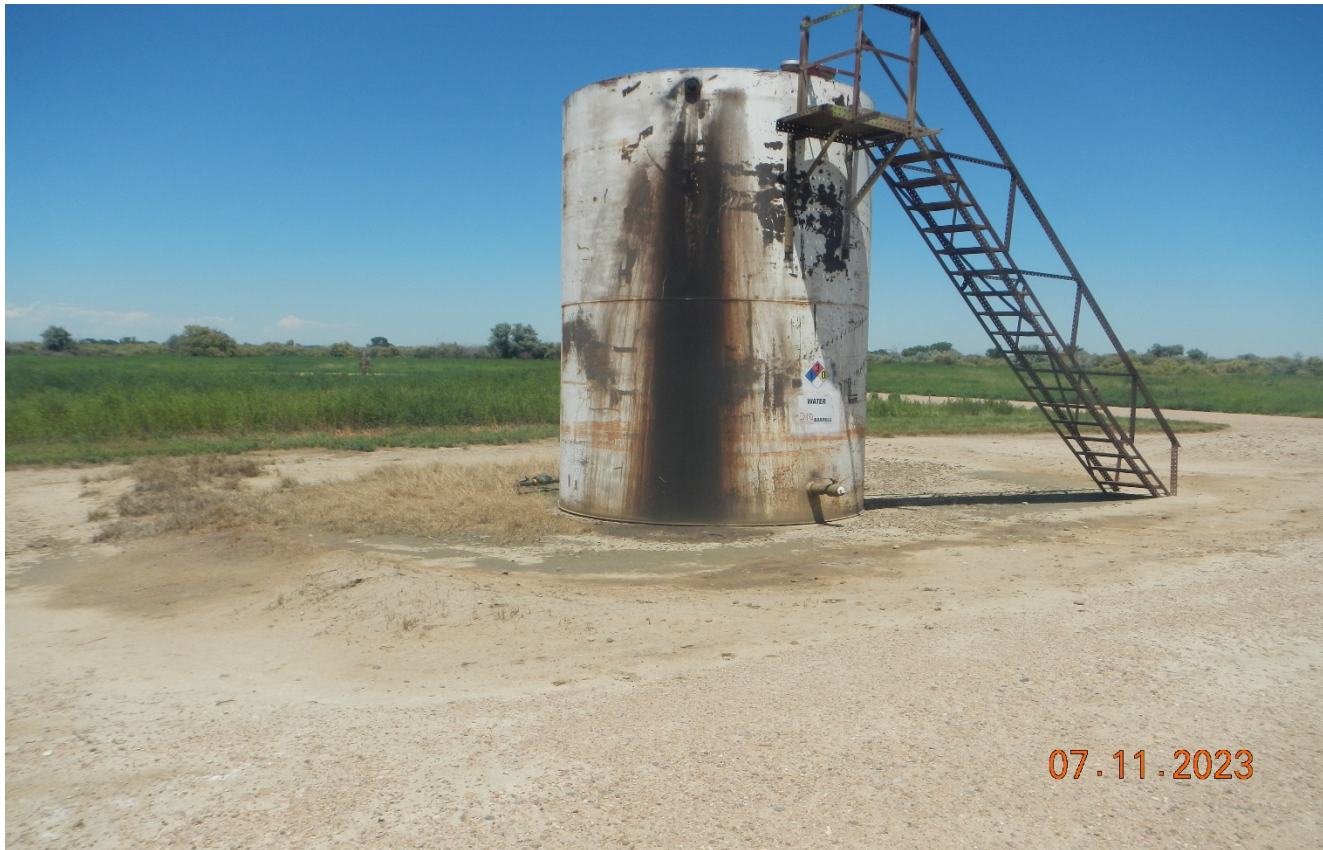
Photo 2. Facing toward the tank which is labeled as water. It appears crude oil has leaked out from the top. Additionally there is no secondary containment around the tank.
