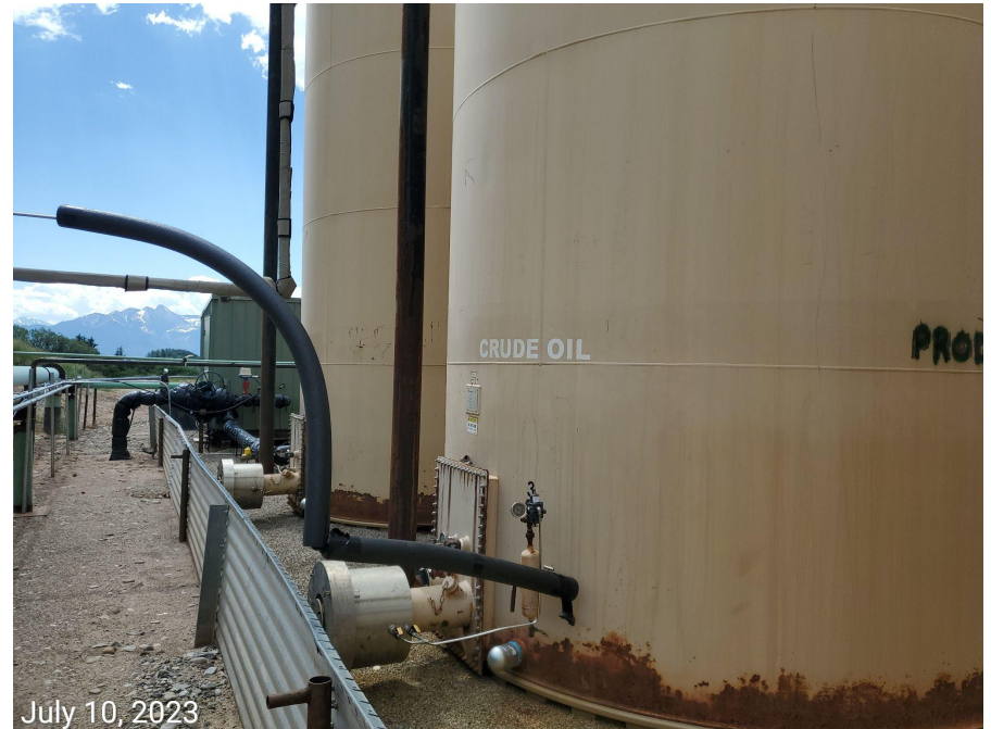
Photo 8: Tank “#3” labeled as both “produced water” and “crude oil”.
