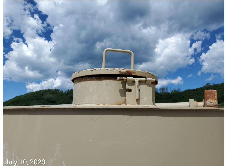
Photo 12: Hatch at the “sand can” not properly secured/closed.
