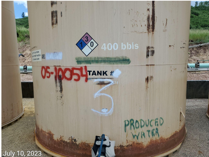
Photo 8: Tank “#3” labeled as both “produced water” and “crude oil”.
