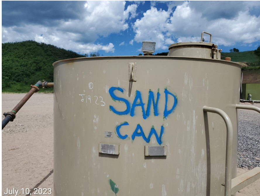
Photo 12: Hatch at the “sand can” not properly secured/closed.
