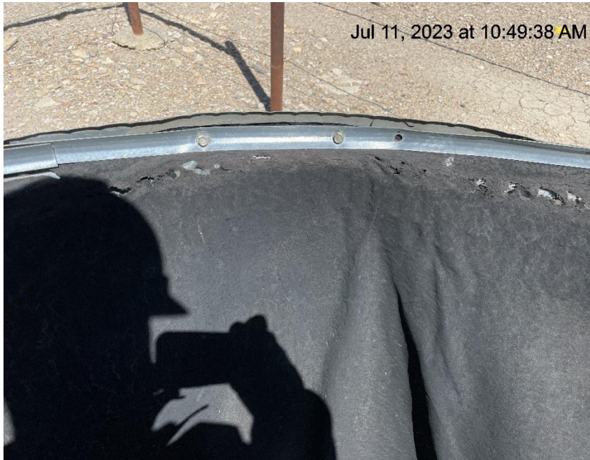
Photo # 2769 Containment liner needs maintenance
