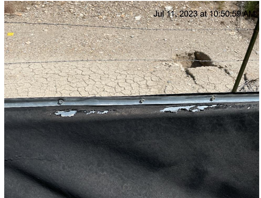
Photo # 2774 Containment needs maintenance
