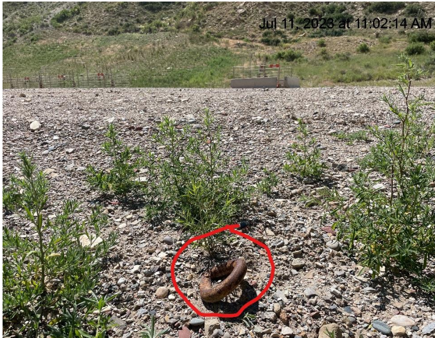
Photo # 2783 Unmarked deadman (N/NW edge of location)
