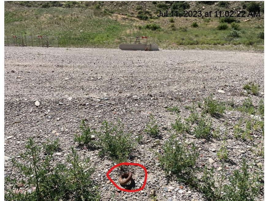
Photo # 2784 Same unmarked deadman from different view
