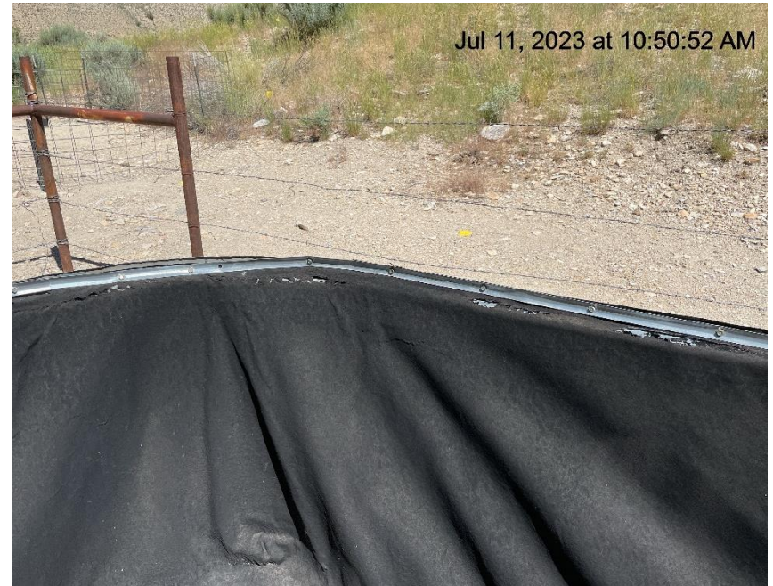
Photo # 2772 Containment liner needs maintenance
