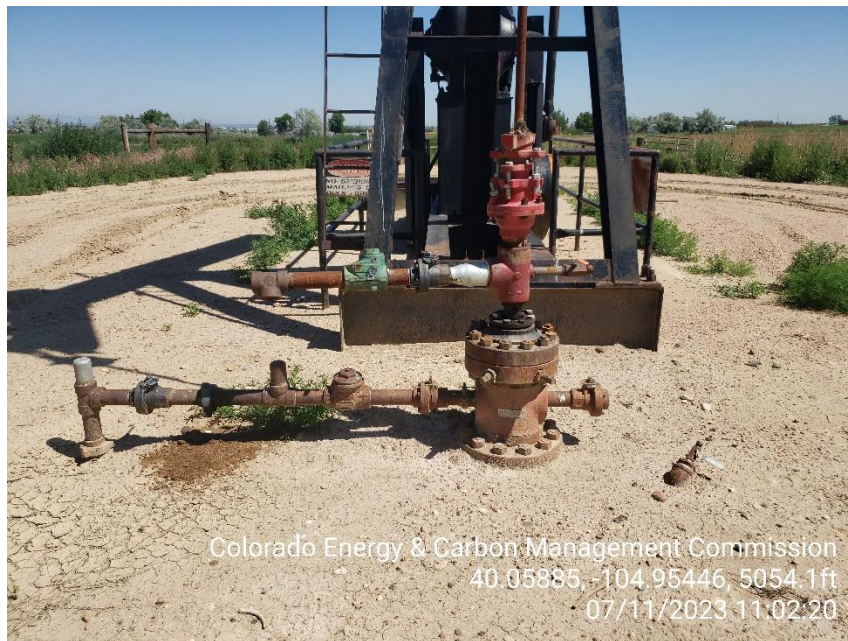
Photo 3 WH, Stained soil under flow line
