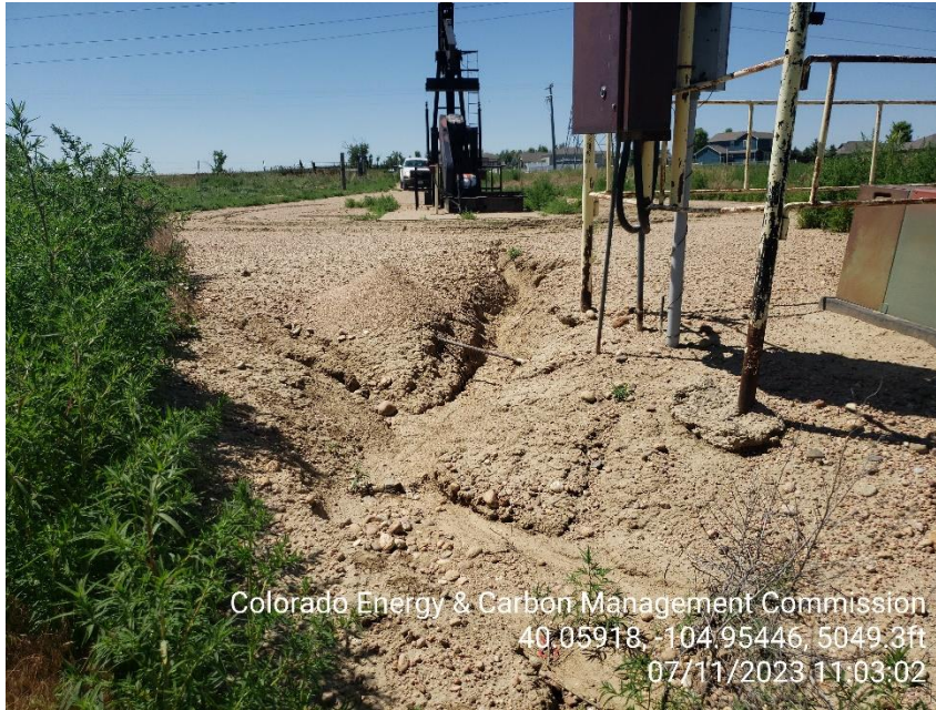
Photo 7 Sediment laden storm water has discharged sediment off location by the ancillary equipment.
