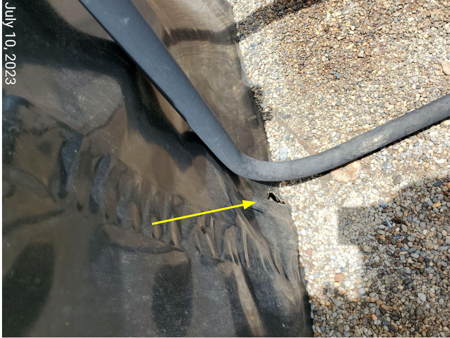
Photo 7: Photos examples showing holes/tears observed within the liner of the tank battery facility's secondary containment BMPs.
