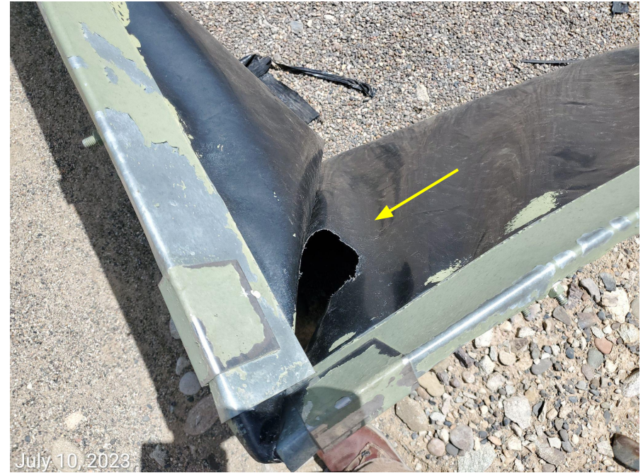
Photo 7: Photos examples showing holes/tears observed within the liner of the tank battery facility's secondary containment BMPs.
