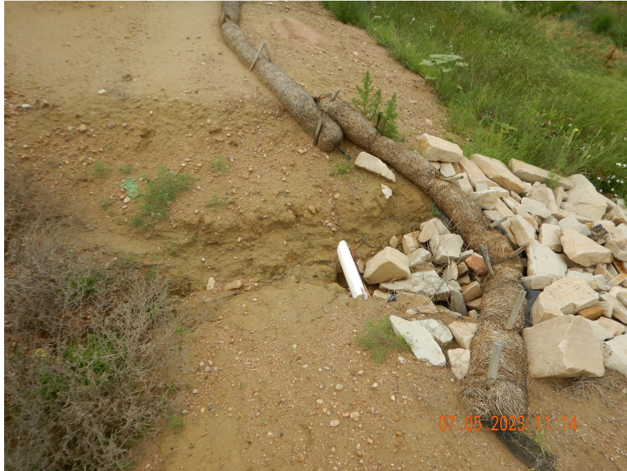
Photo 4. Photo taken from the eastern location. Photo illustrates stormwater BMPs have been installed but are in need of repair. Gully erosion is exposing an unknown line.
