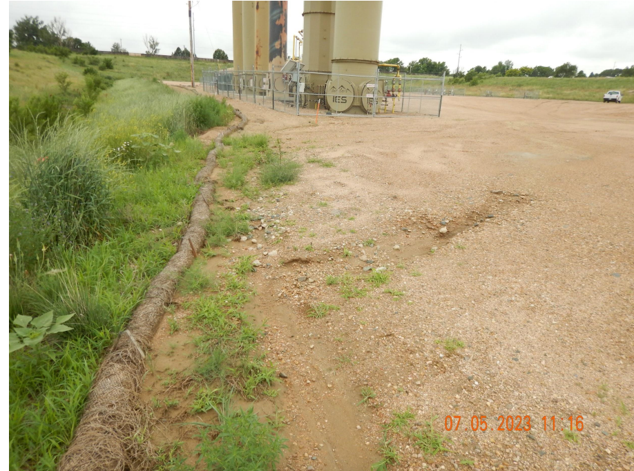
Photo 5. Photo taken from the northeastern location, facing South. Photo illustrates a stormwater BMP in need of repair, as sediment has discharged off location and beyond the BMP. Refer to Photo 6.
