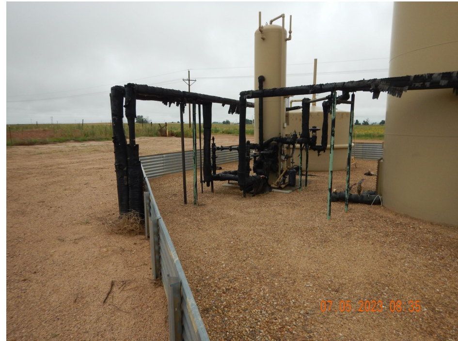
Photo 6. Photo taken from the associated offsite tank battery. Photo illustrates tape that is degrading. Tape and foam coming off piping, which is contributing to trash around the location.
