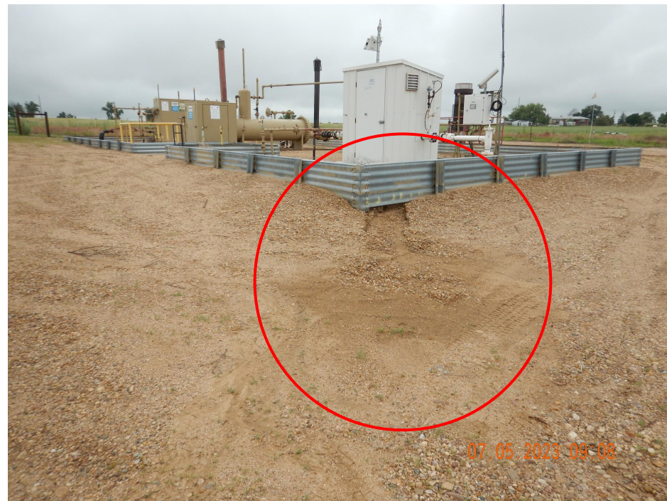
Photo 8. Photo taken from the associated offsite tank battery, facing South. Photo illustrates stormwater erosion that is compromising secondary containment.
