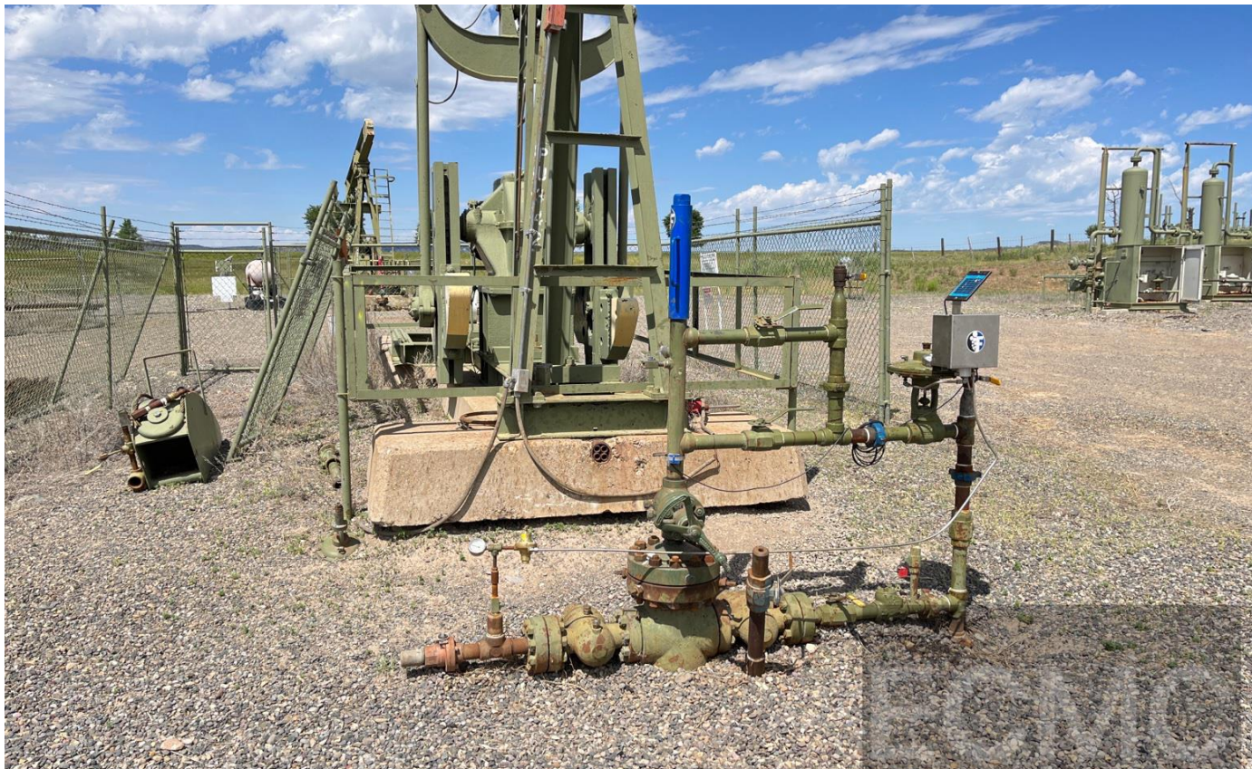
Photo #3. View of the 13-1 wellhead assembly.
