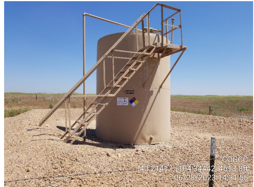
Photo 4 – Tank Battery – Sign Missing
