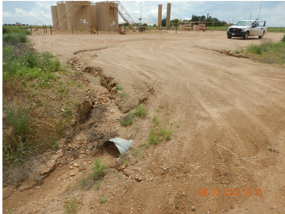
Photo 2. Photo taken from the associated offsite tank battery, facing Southwest. Photo illustrates gully erosion without sufficient stormwater BMPs. Also, the culvert is in need of repair.
