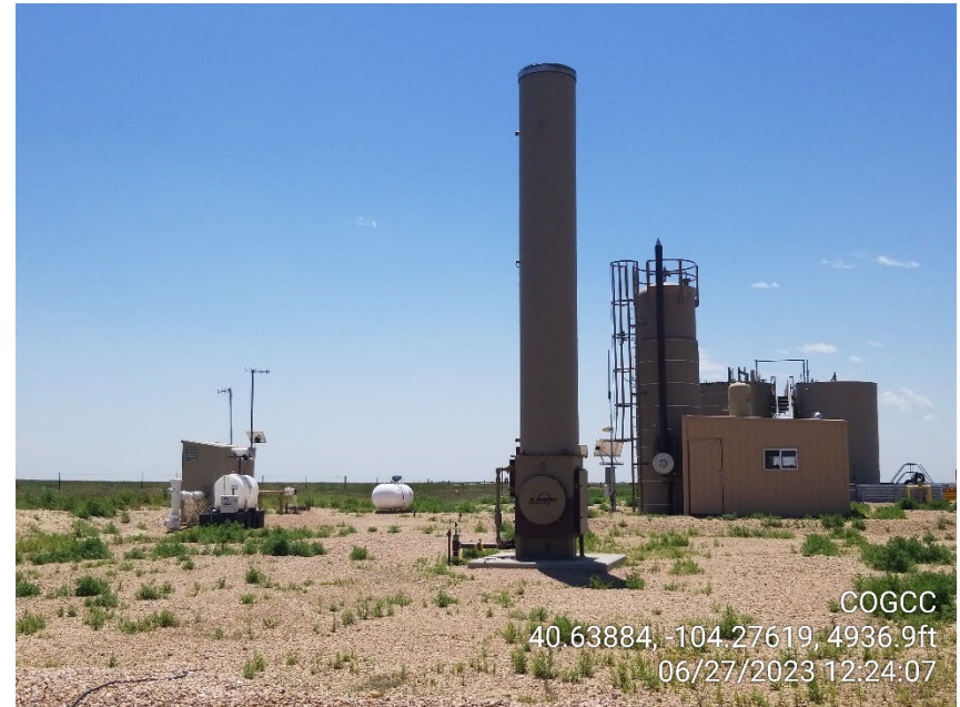
Photo 8 – ECD, Gas Meter and Heater Treater
