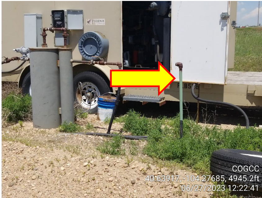
Photo 3 – Generator – Unmarked Riser
