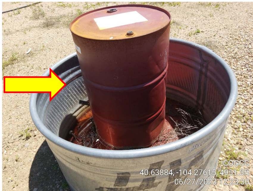
Photo 5 – Containment – Wildlife Netting missing and Debris inside Containment
