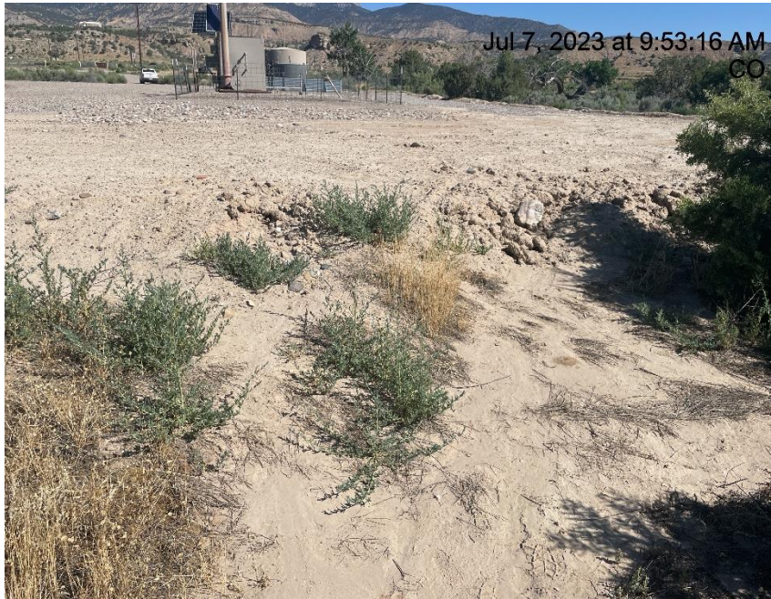
Photo # 2473 Erosion & transport of sediment off location & into vegetated area
