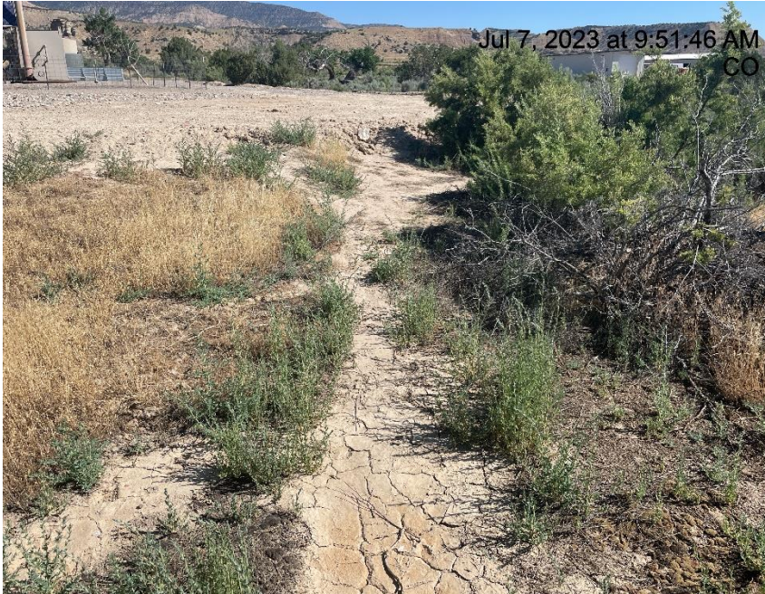
Photo # 2468 Erosion & transport of sediment off location & into vegetated area
