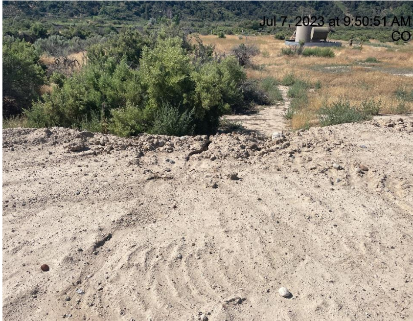
Photo # 2463 Erosion & transport of sediment off location & into vegetated area
