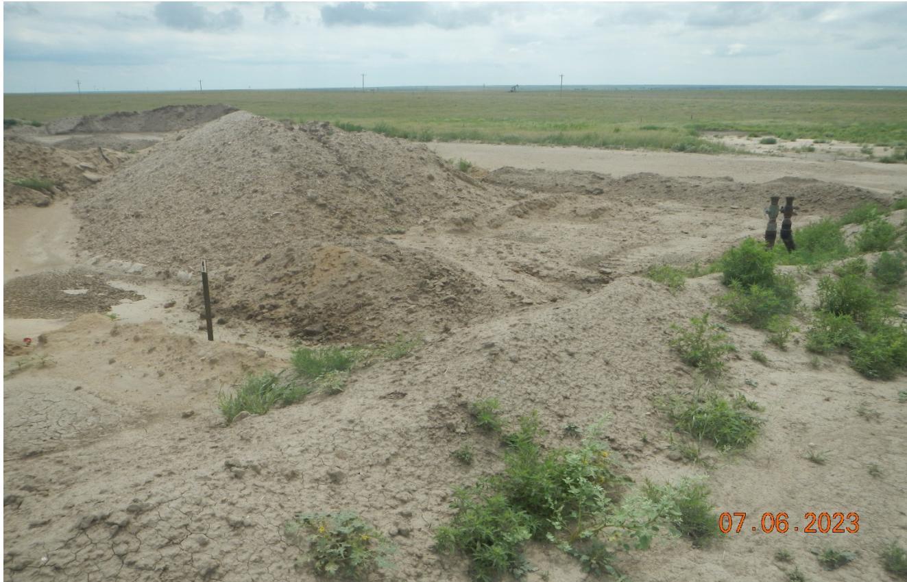
Photo 2. Facing southwest toward the tank battery facility. The tank was removed and soils were excavated in this area. It appears soils have been backfilled into the excavated area where tanks were located. There is still a pile of contaminated material improperly stored at the location.
