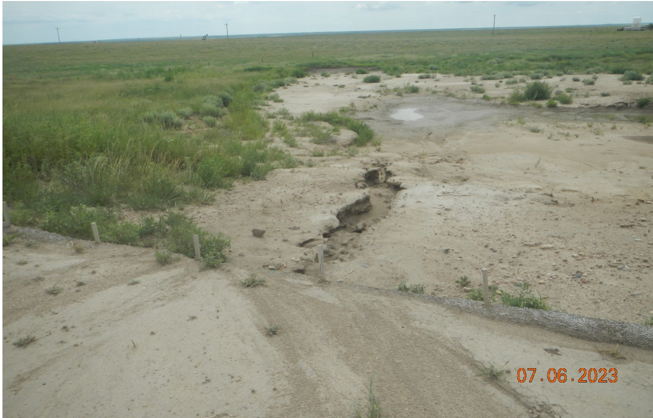
Photo 5. View of wattles which sediment has filled in and overtopped moving sediment offsite causing additional erosion.
