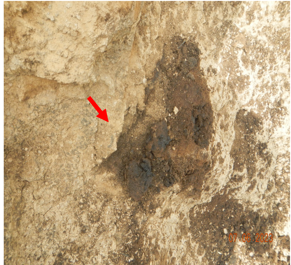
Photo 9. Located at the western side of the spill area. There is an excavated hole at this area approximately 12'x12'6'. There are still areas of oil stained soils at the surface (Bottom left) and 2ft. Down into the excavation area (right photo). Further excavation is needed.
