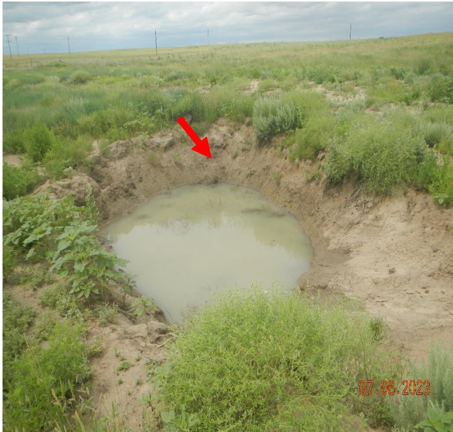
Photo 9. Located at the western side of the spill area. There is an excavated hole at this area approximately 12'x12'6'. There are still areas of oil stained soils at the surface (Bottom left) and 2ft. Down into the excavation area (right photo). Further excavation is needed.
