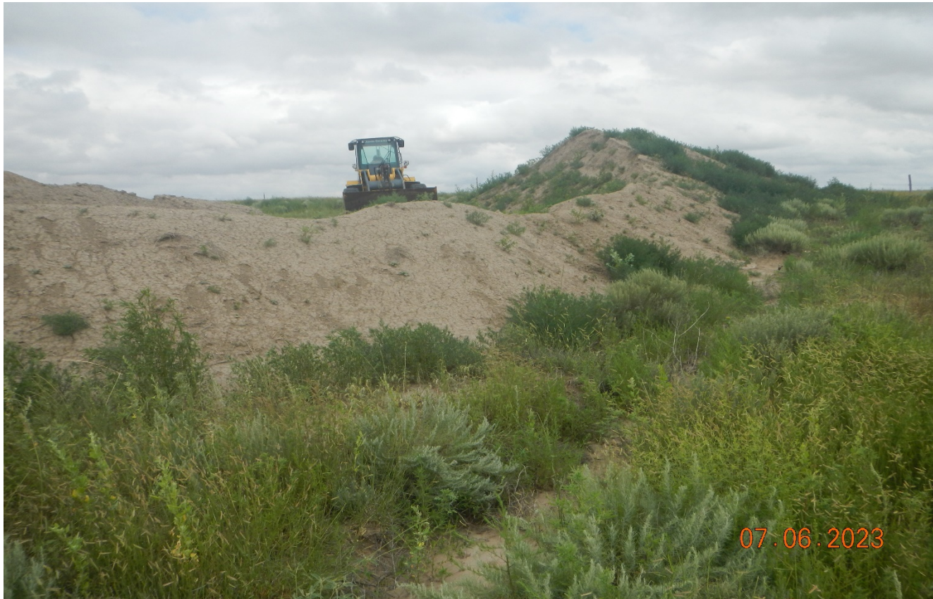
Photo 6. There have been soils brought in and stockpiled at the south side of the location. There is inadequate stormwater BMP's to prevent erosion of the stock piled soil. Previous corrective action was not completed.
