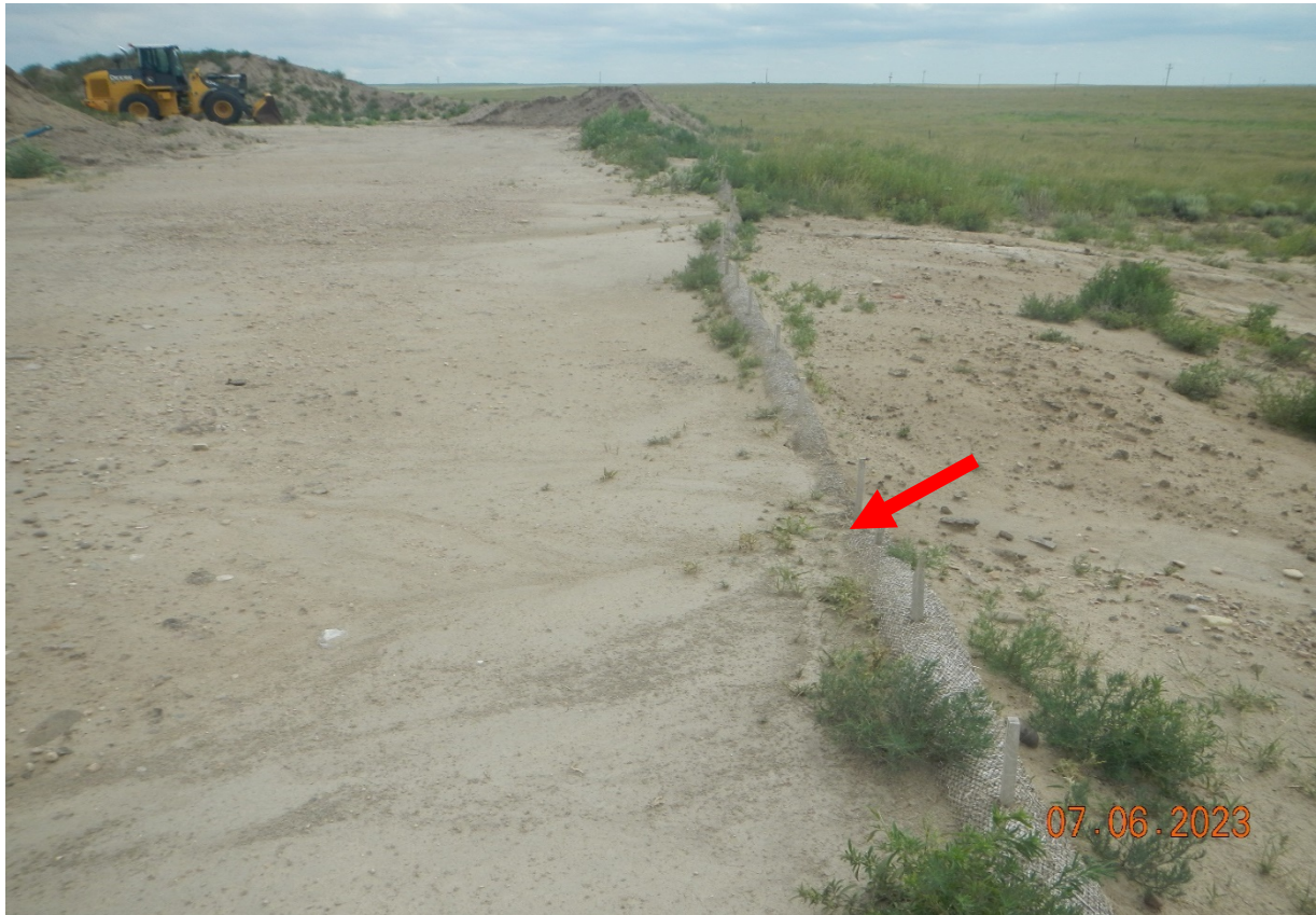
Photo 4. Facing south at the tank battery facility. There is insufficient stormwater controls in this area and the wattles at red arrow have filled with sediment which has overtopped the wattles.
