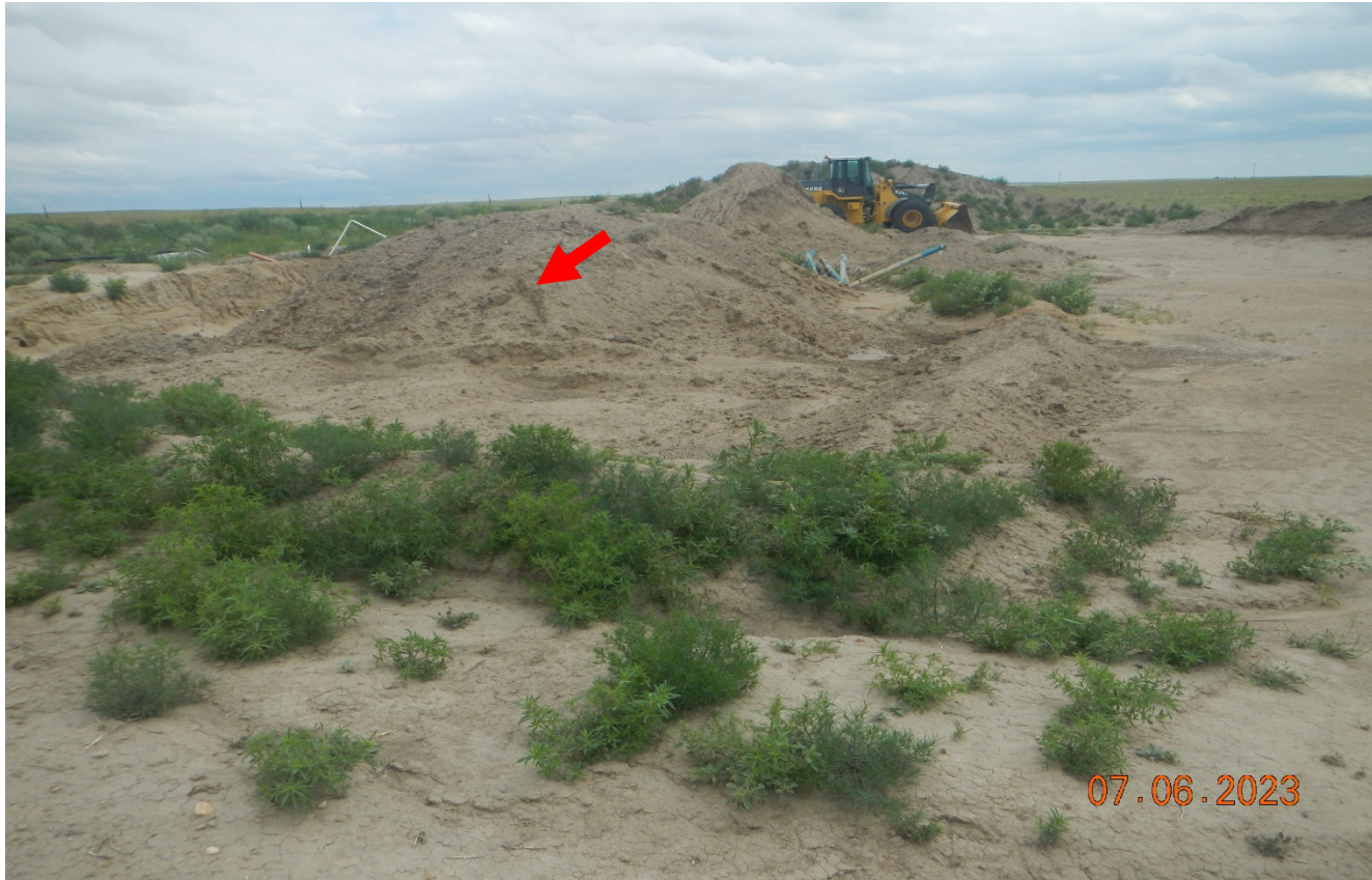
Photo 3. There is no liner observed under the contaminated soils which are not being properly stored. The berms around the material are not compacted or adequately constructed. Contaminated soils need to be removed and properly disposed. Red arrow points to black hydrocarbon soils.
