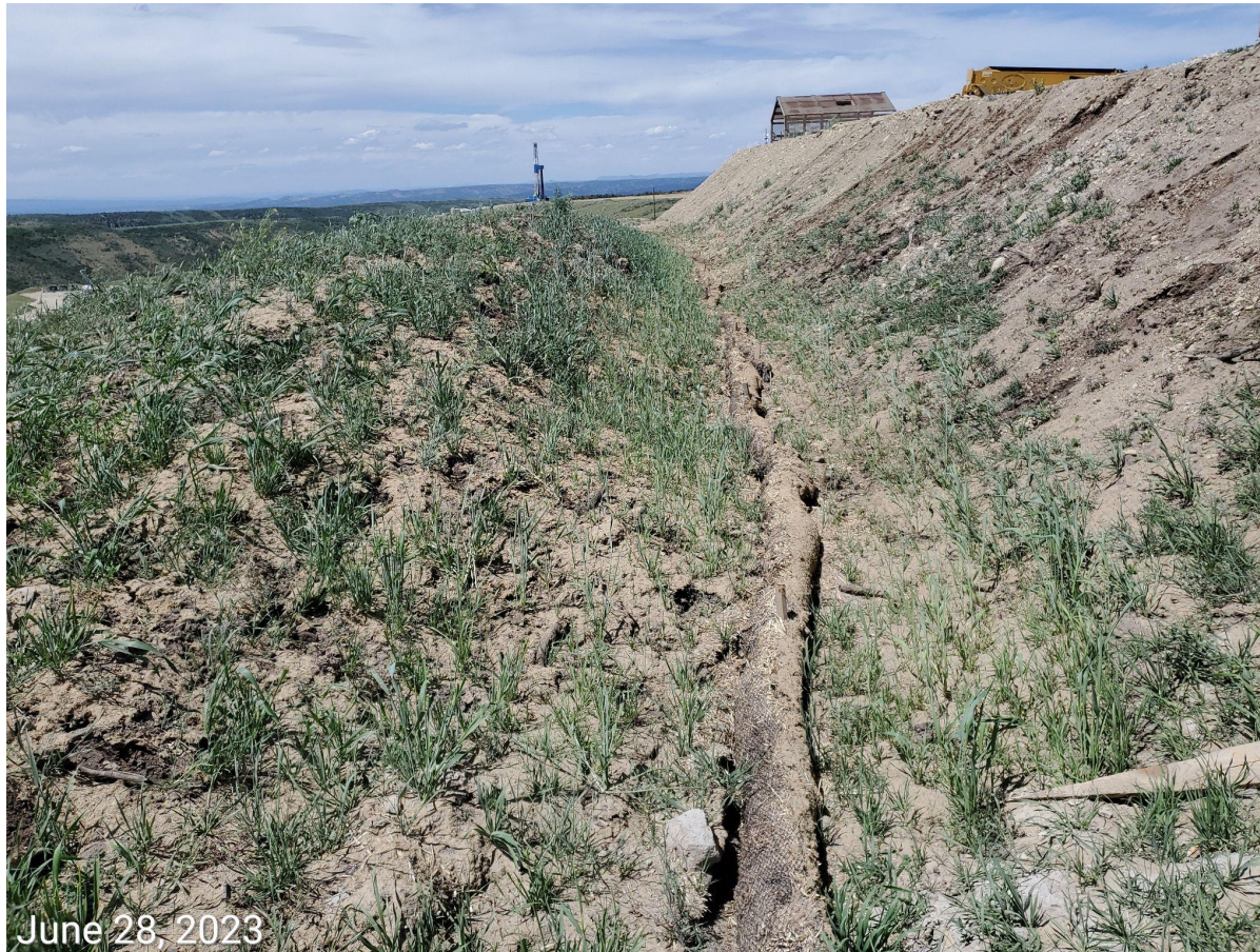
Photo 27: Photos 27-28 taken from the topsoil stockpiles on the perimeter of the Location. Photos show Operator has implemented additional BMPs to protect the topsoil stockpiles, and to ensure soils remain properly segregated, and not incorporated as part of stormwater management BMPs for the Location.
