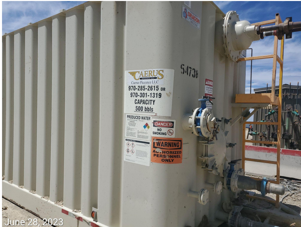
Photo 20: Photo example of tank on the Location with required label information including, but not limited to, Operator name, emergency contact number, tank capacity, tank contents, NFPA label, etc... Photos also shows tank is missing spill prevention/containment BMPs.
