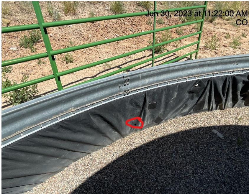
Photo # 2271 Hole in secondary containment liner/liner needs maintenance
