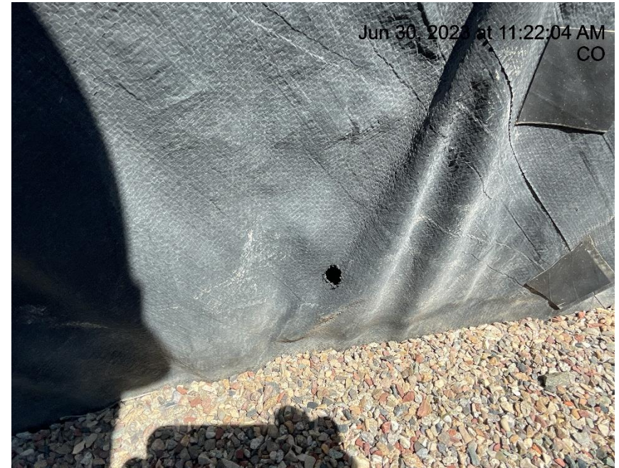
Photo # 2272 Hole in secondary containment liner/liner needs maintenance
