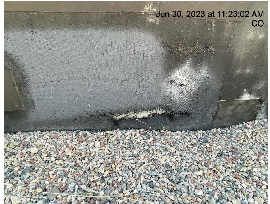
Photo # 2282 Hole in secondary containment liner/liner needs maintenance
