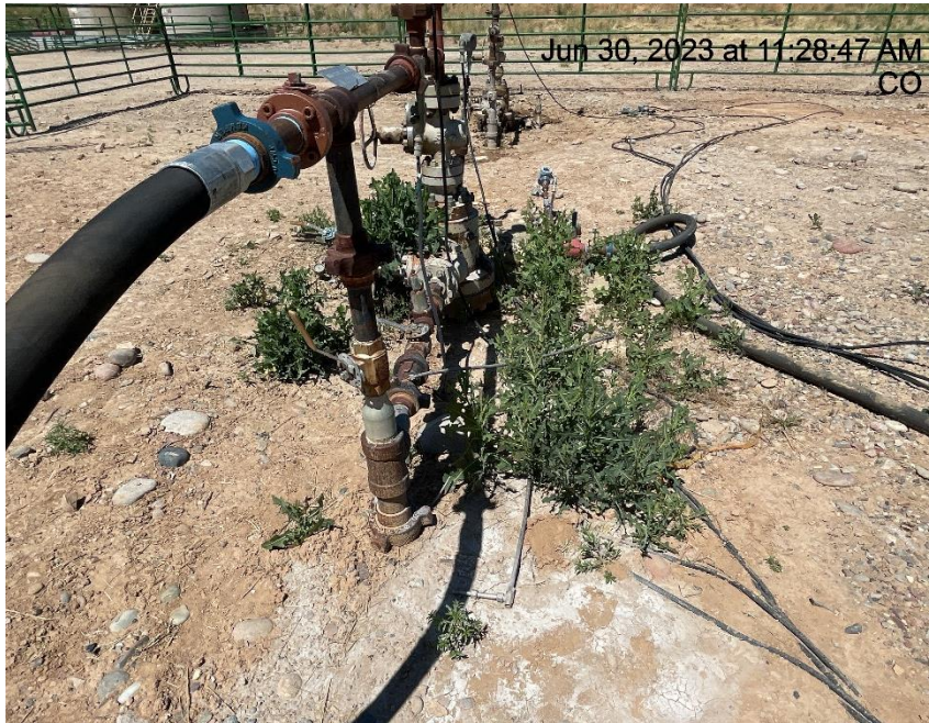
Photo # 2304 KELLY 34-13 well bradenhead connected to flowline, no check valve visible
