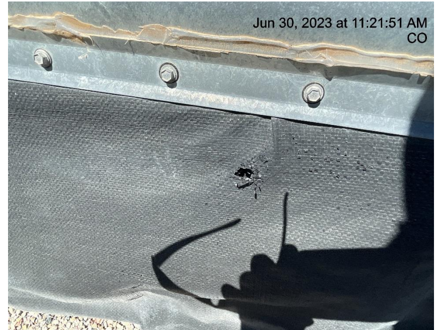
Photo # 2270 Hole in secondary containment liner/liner needs maintenance
