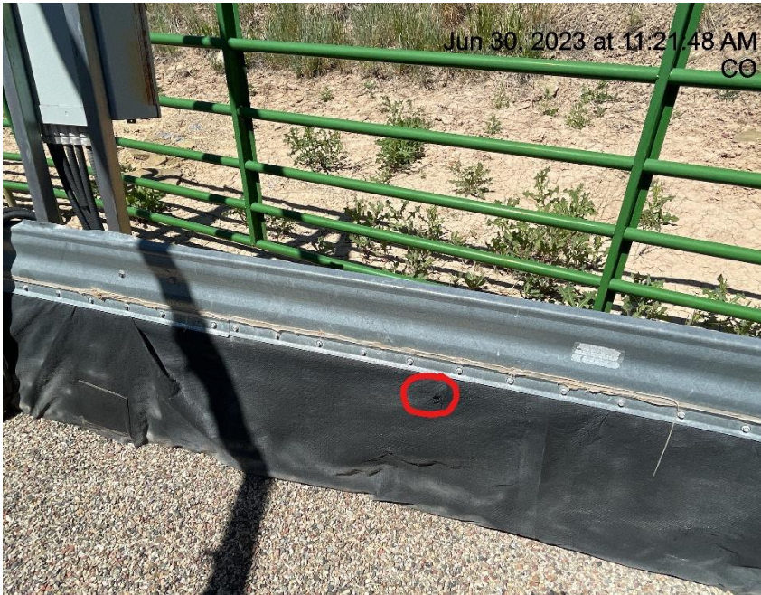
Photo # 2269 Hole in secondary containment liner/liner needs maintenance
