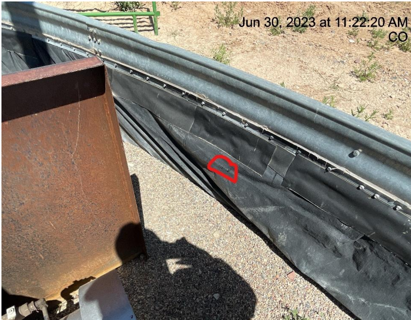
Photo # 2275 Hole in secondary containment liner/liner needs maintenance
