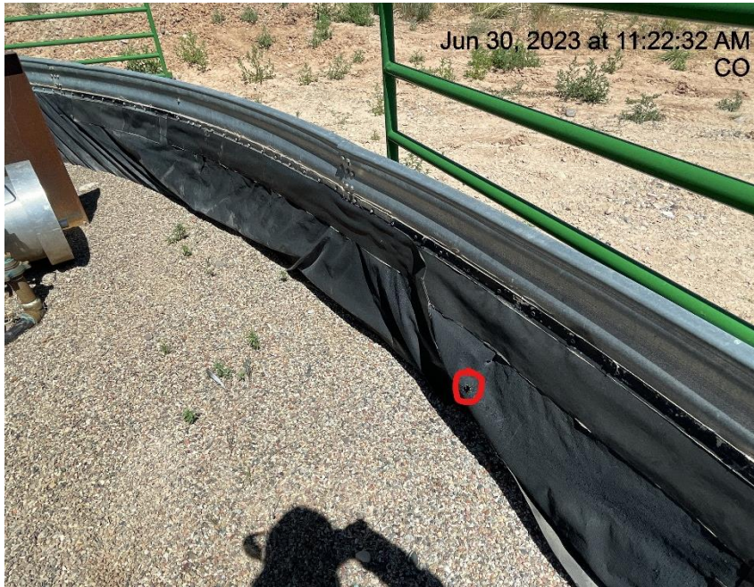
Photo # 2277 Hole in secondary containment liner/liner needs maintenance
