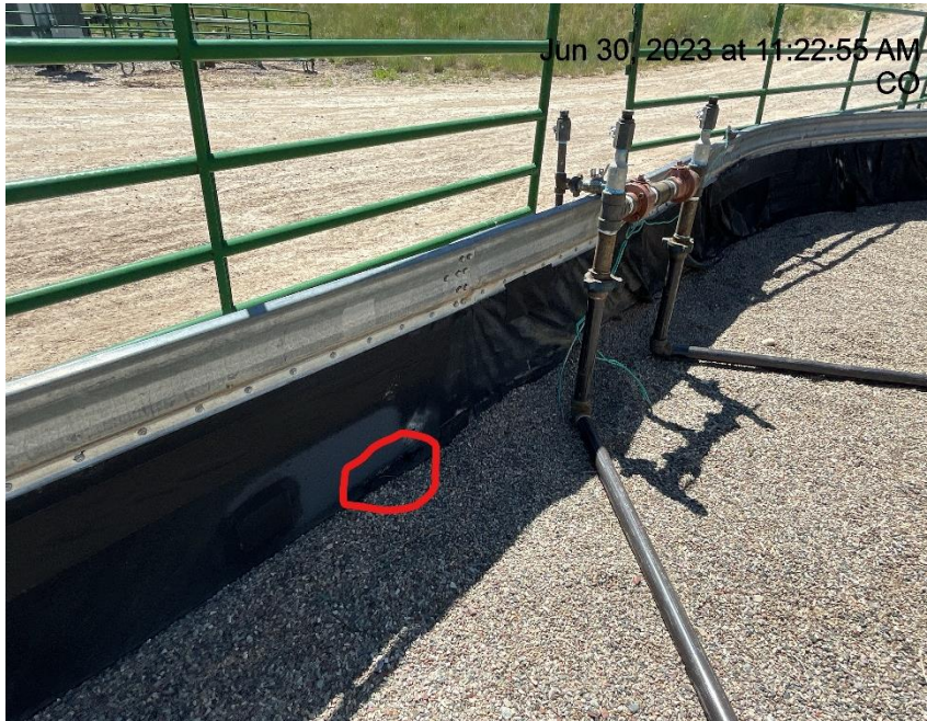
Photo # 2281 Hole in secondary containment liner/liner needs maintenance
