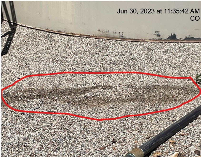
Photo # 2316 Stained gravel inside secondary containment
