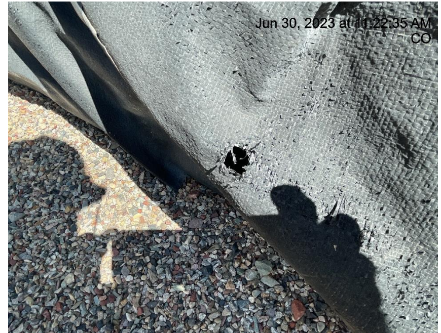
Photo # 2278 Hole in secondary containment liner/liner needs maintenance
