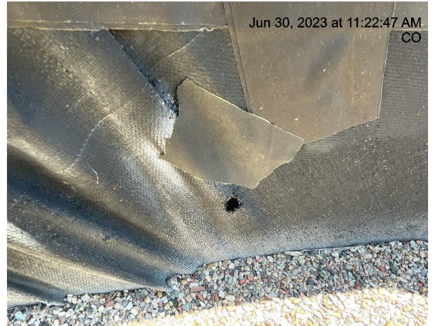
Photo # 2280 Hole in secondary containment liner/liner needs maintenance
