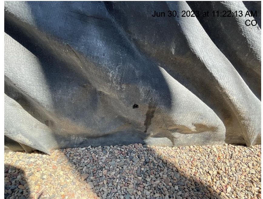
Photo # 2274 Hole in secondary containment liner/liner needs maintenance
