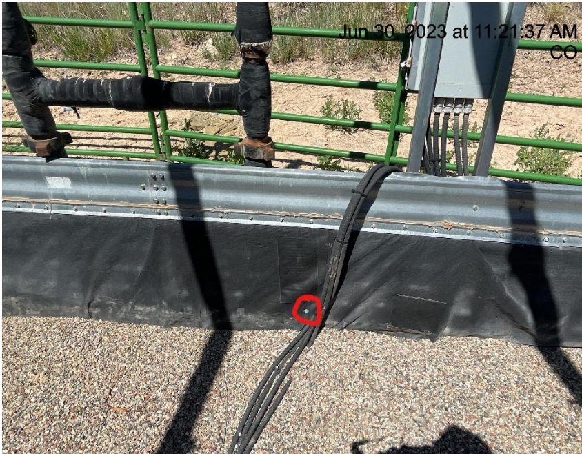
Photo # 2267 Hole in secondary containment liner/liner needs maintenance
