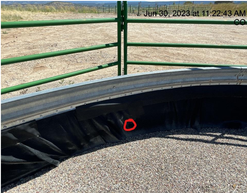
Photo # 2279 Hole in secondary containment liner/liner needs maintenance
