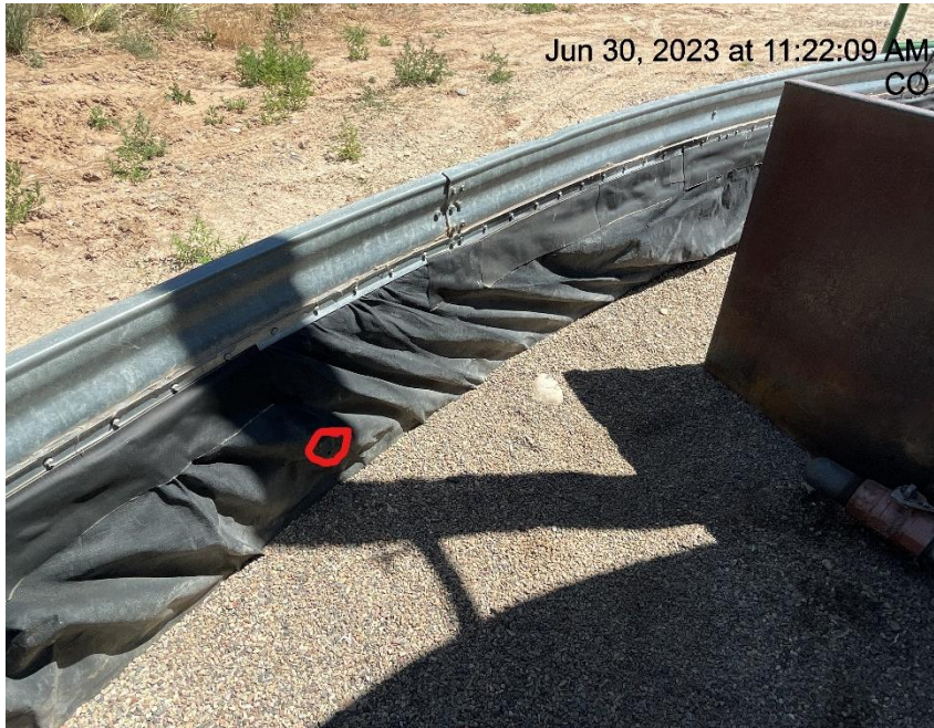
Photo # 2273 Hole in secondary containment liner/liner needs maintenance
