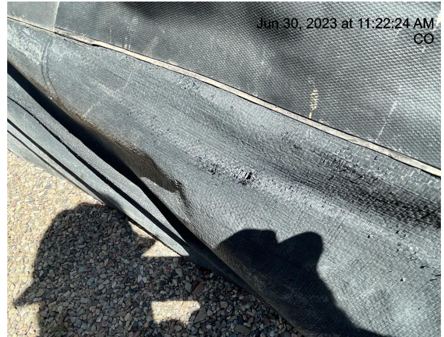
Photo # 2276 Hole in secondary containment liner/liner needs maintenance
