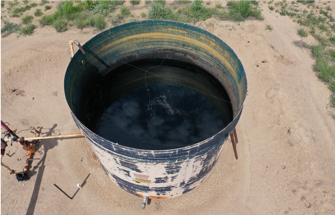
Photo 7. Drone photo looking down at the open top tanks shows no netting over the tank. Tank is approximately \frac{3}{4} full of crude oil.
