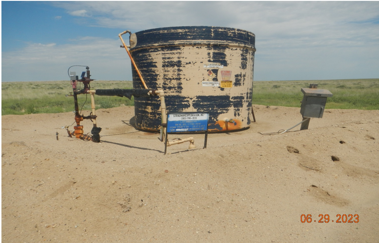
Photo 6. Facing toward the wellsite. The labeling on the tank is faded and peeled off. There is animal burrows in the secondary containment berm which needs t be repaired.
