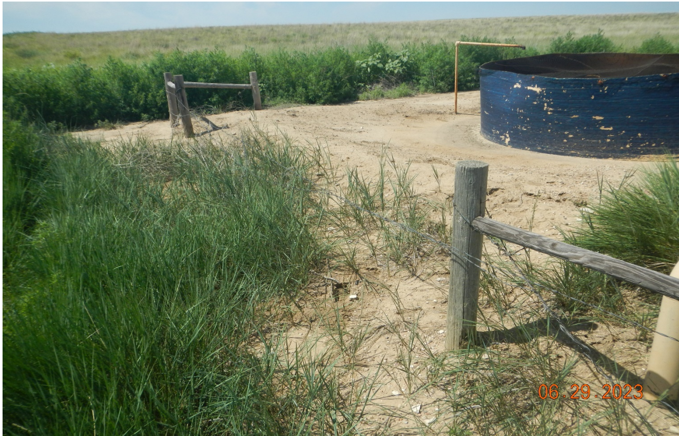
Photo 4. The fence around the open top tank is inadequate to prevent livestock entry and is not maintained. The berm around the tank is insufficient to contain a spill.
