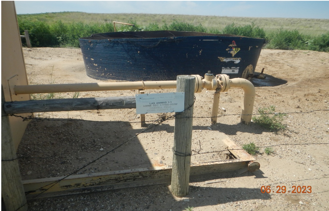
Photo 5. The offsite tank battery sign is faded and does not meet the signage requirement of rule 605.
