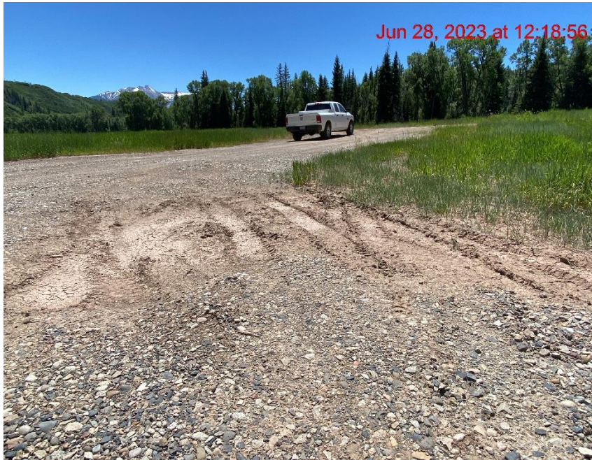
Location Lacks Stabilization – Photo #04906
