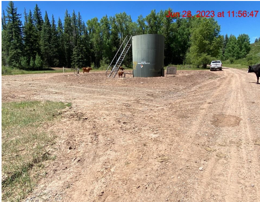
Insufficient Vehicle Tracking BMPs at Location Entrance/Exit – Photo #04880
