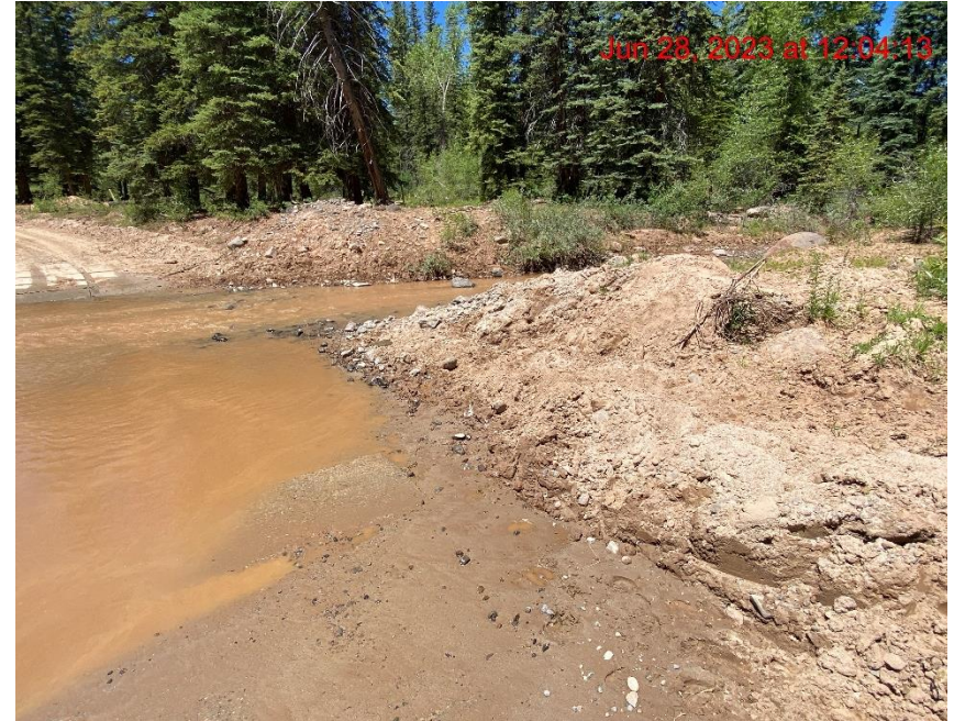
Unprotected Spoil Piles Near Creek on Lease Road – Photo #04886
