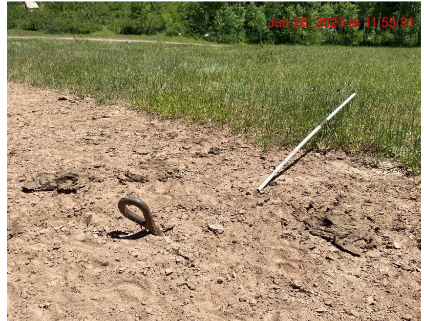
Anchor not Adequately Marked– Photo #04877
