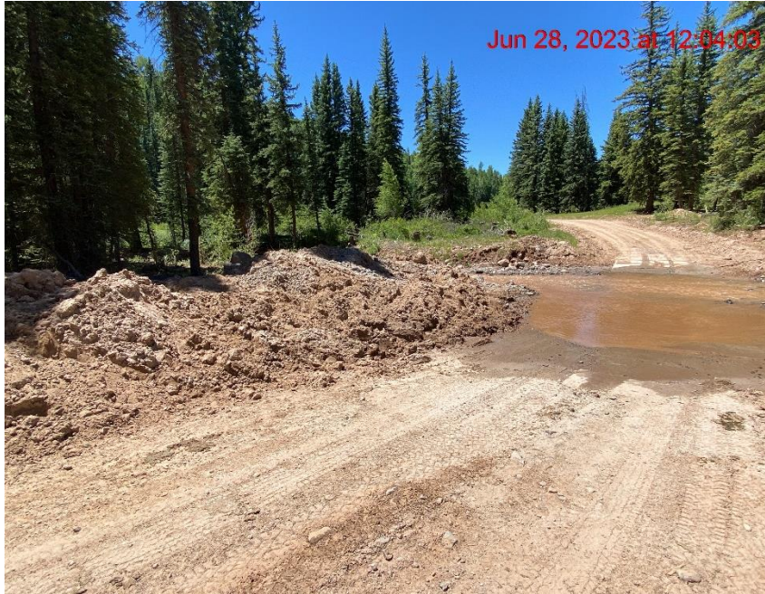
Unprotected Spoil Piles Near Creek on Lease Road – Photo #04885
