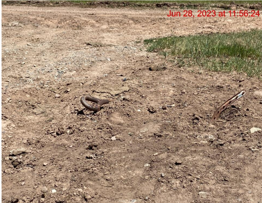
Anchor not Adequately Marked – Photo #04879
