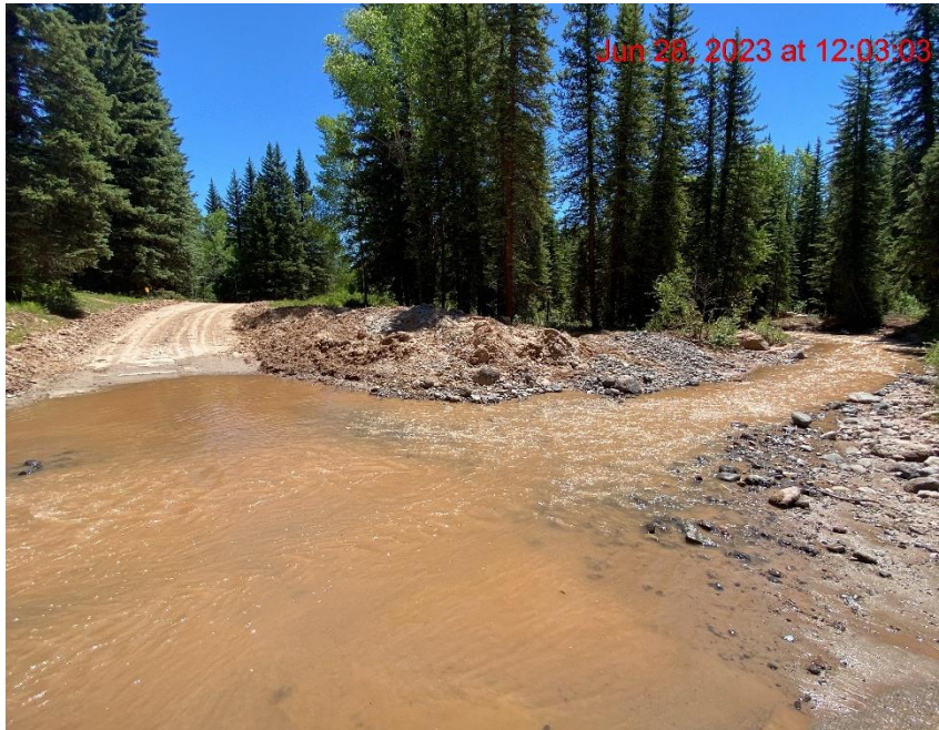
Unprotected Spoil Piles Near Creek on Lease Road – Photo #04883
