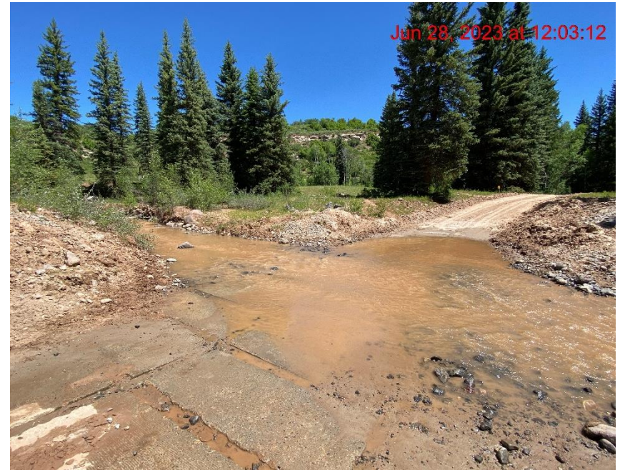
Unprotected Spoil Piles Near Creek on Lease Road – Photo #04884
