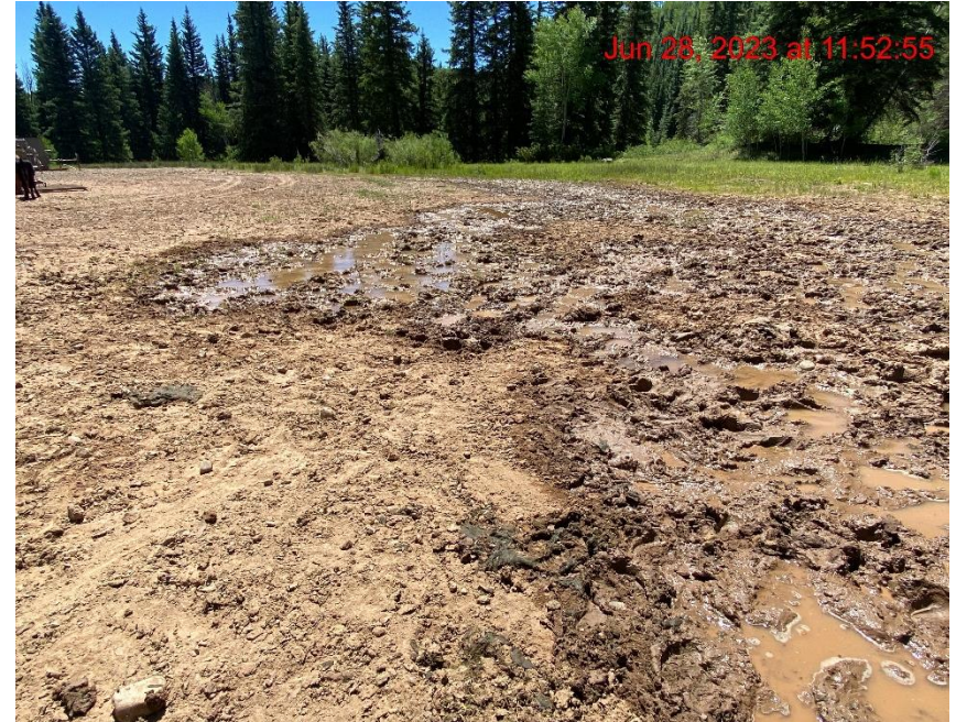
Location Lacks Stabilization – Photo #04870
