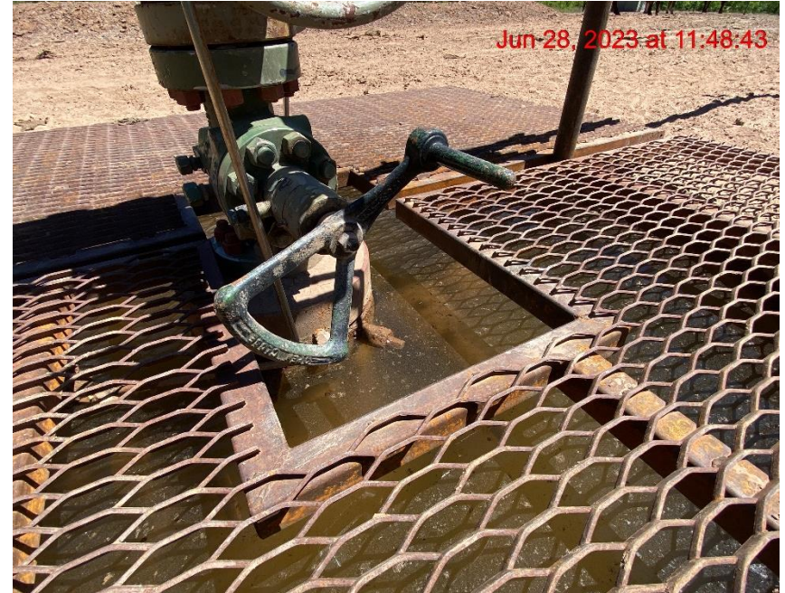
Wellhead Cellar Full of Water – Photo #04859
