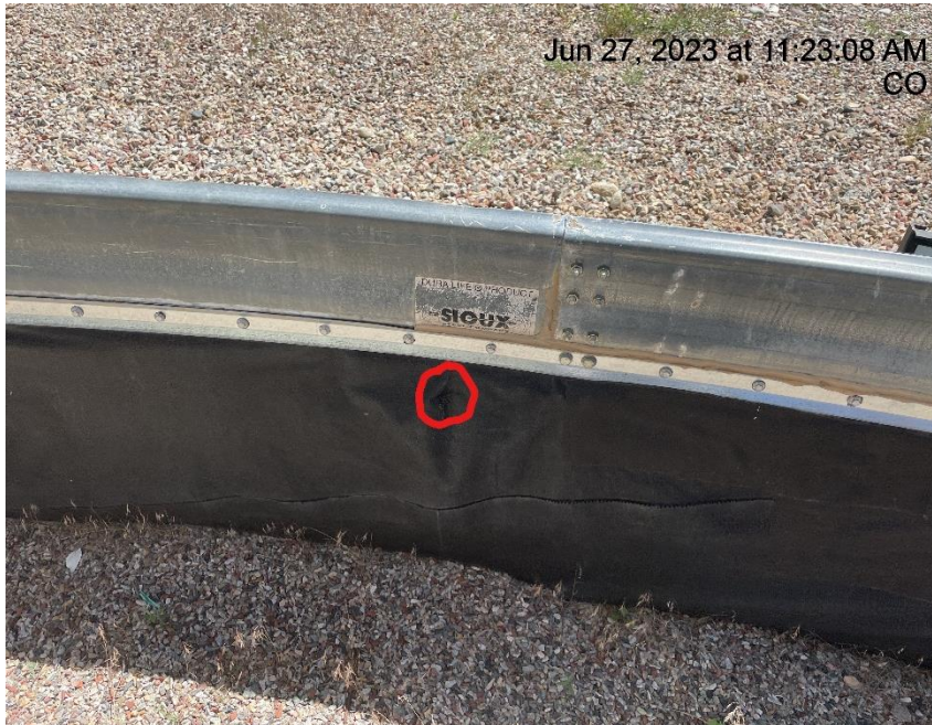
Photo # 2105 Hole in liner/liner needs maintenance
