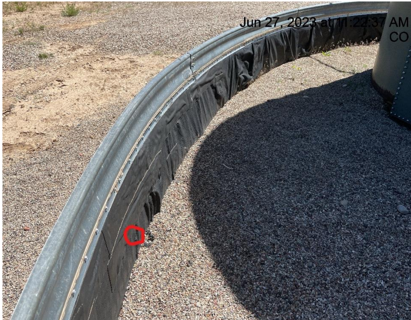
Photo # 2103 Hole in liner/liner needs maintenance
