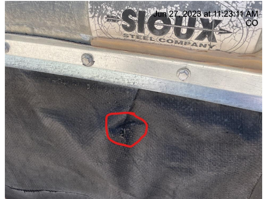
Photo # 2106 Hole in liner/liner needs maintenance
