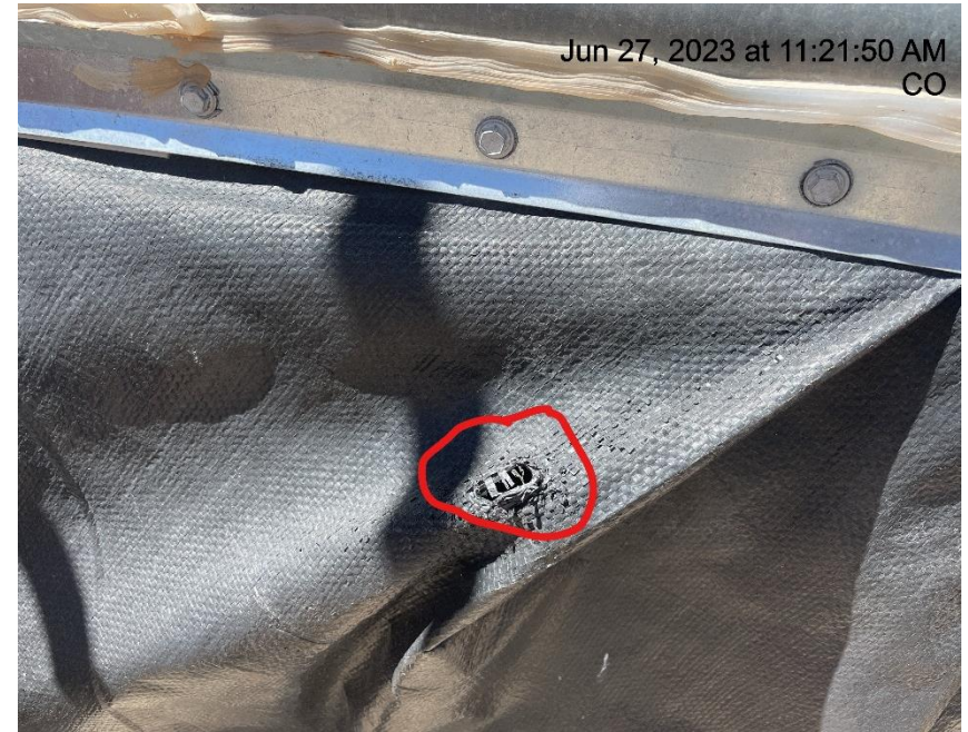
Photo # 2102 Hole in liner/liner needs maintenance
