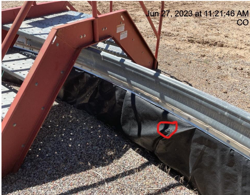
Photo # 2101 Hole in liner/liner needs maintenance
