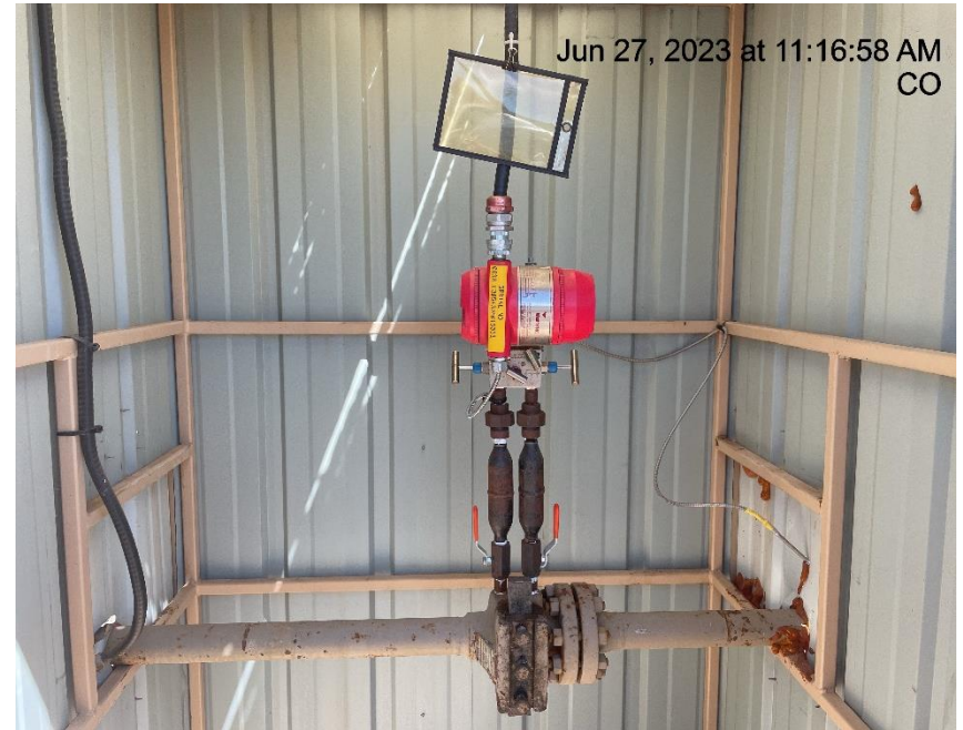
Photo # 2093 COUEY 17-14 well missing calibration info/Meter calibration info not conspicuously posted
