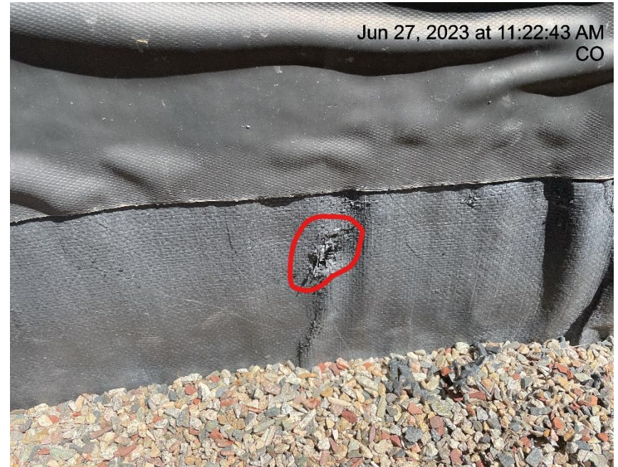
Photo # 2104 Hole in liner/liner needs maintenance
