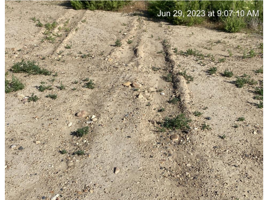
Stormwater BMPs not in place
