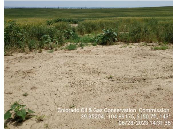
**Photo 5 No BMPs installed, sediment is washing off the wellsite into the planted field towards the SE.**
