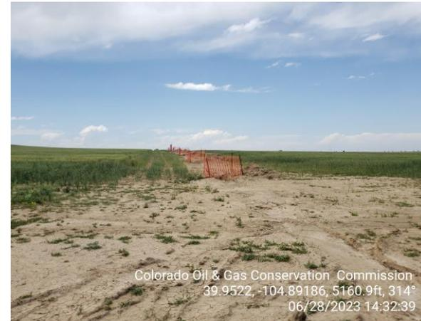
**Photo 8 Flow line excavation looking to the battery, sediment is running off into the planted field.**
