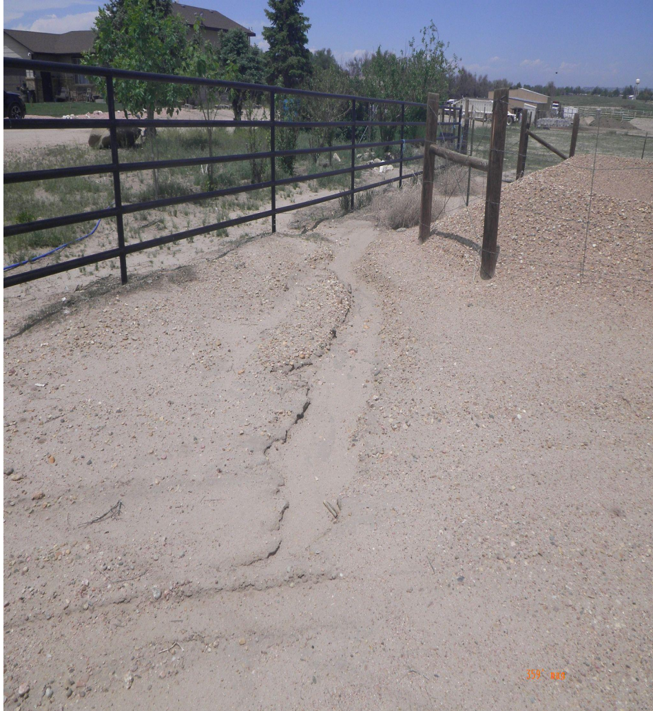
Photo 3. Rill erosion observed on the western edge of the tank battery has not been addressed since previous inspection form was submitted on November 16th, 2021.
