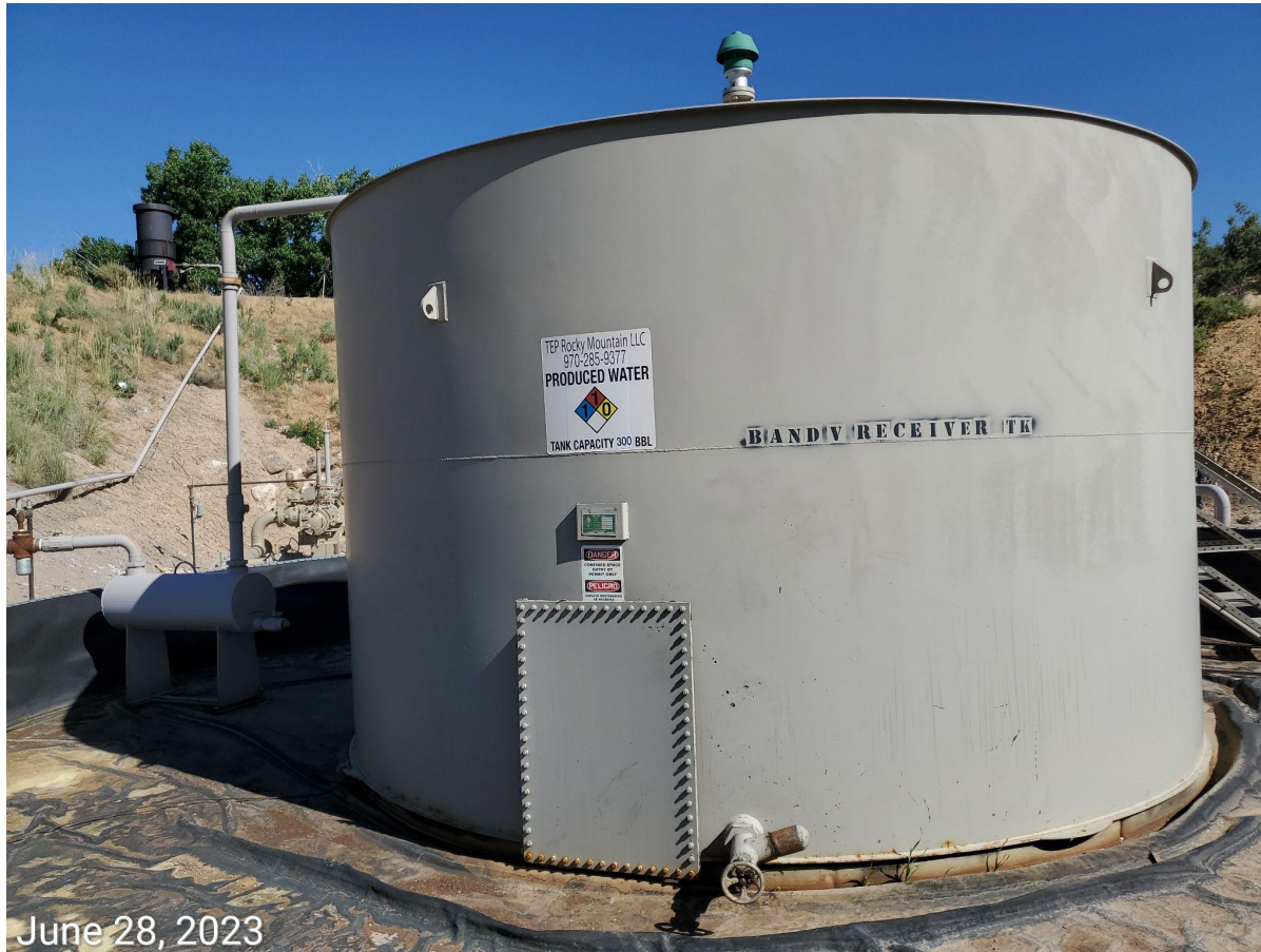
Photo 16: Photo shows tank battery on the west end of the Location. Signage required per Rule 605.e not observed at facility.
