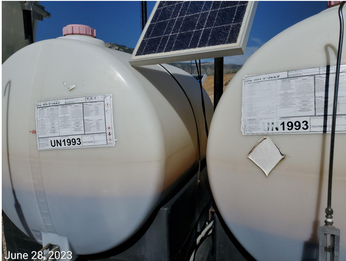
Photo 17: Labels at methanol tanks becoming illegible. Maintenance advised.
