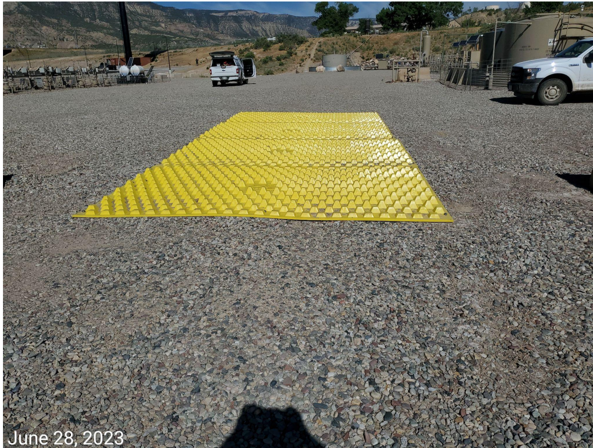
Photo 7: Vehicle tracking pad
