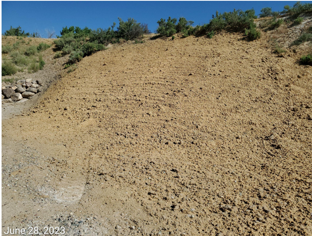
Photo 12: Slopes on northwest end of the Location. Slopes appear to have been recently hydromulched. BMP appears to be in proper functioning condition.
