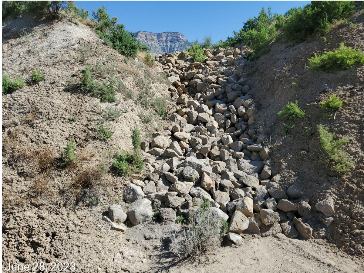
Photo 9: Armored inlet to manage run-on, on the north end of the Location.
