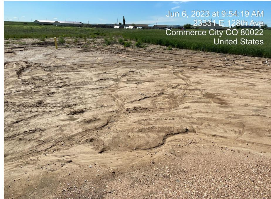
**Photo 4. Photo of erosion on site from recent rains.**
