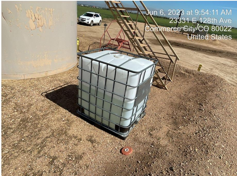
**Photo 3. Photo taken of unlabeled open tote on site. Berm around tanke battery is insufficient.**
