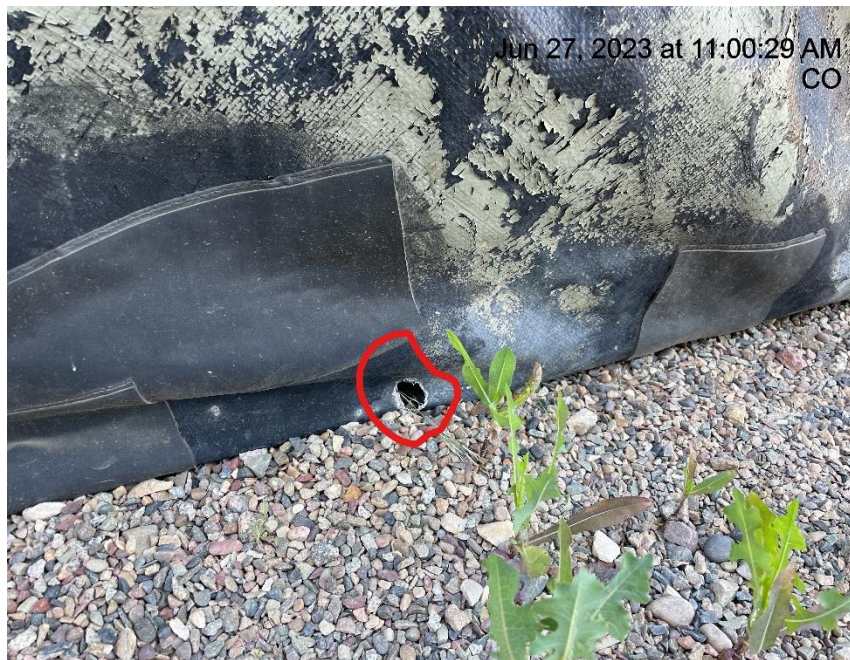
Photo # 2073 Hole in liner/liner needs maintenance
