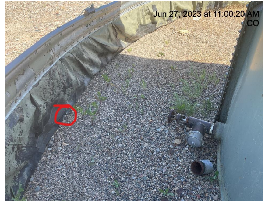
Photo # 2072 Hole in liner/liner needs maintenance
