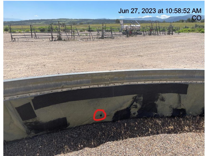
Photo # 2066 Hole in liner/liner needs maintenance
