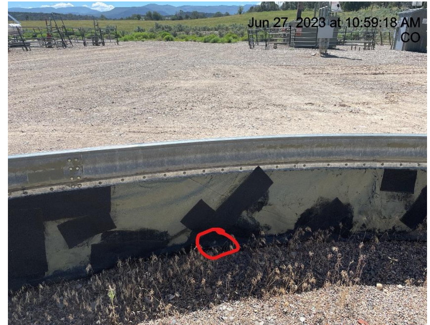
Photo # 2068 Hole in liner/liner needs maintenance
