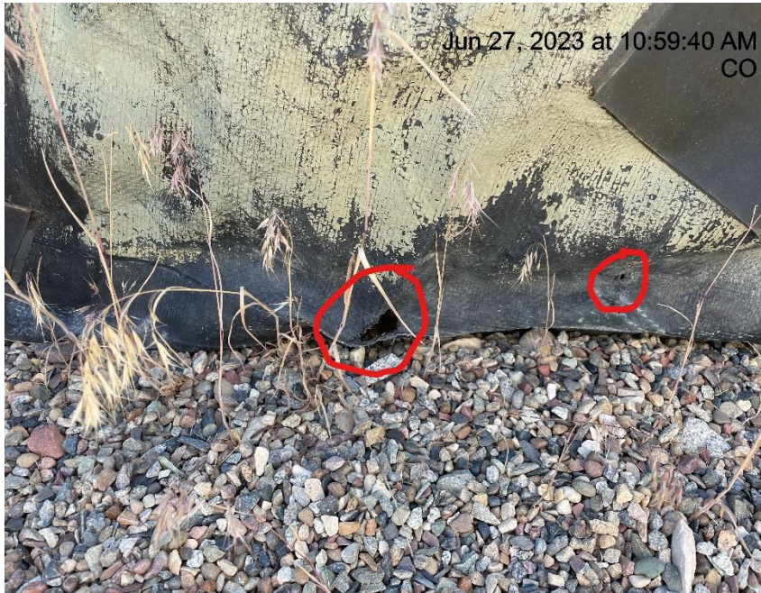
Photo # 2071 Hole in liner/liner needs maintenance
