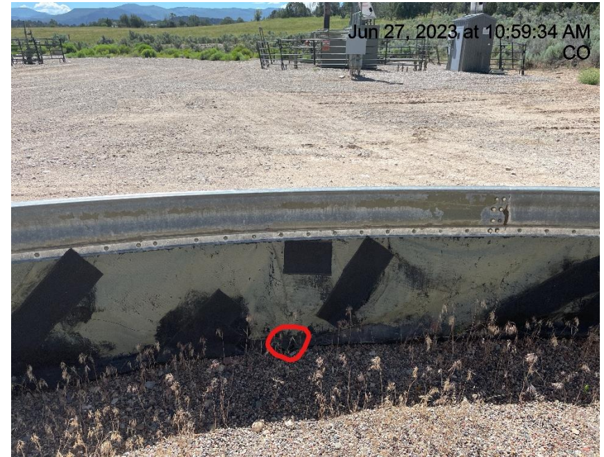
Photo # 2070 Hole in liner/liner needs maintenance
