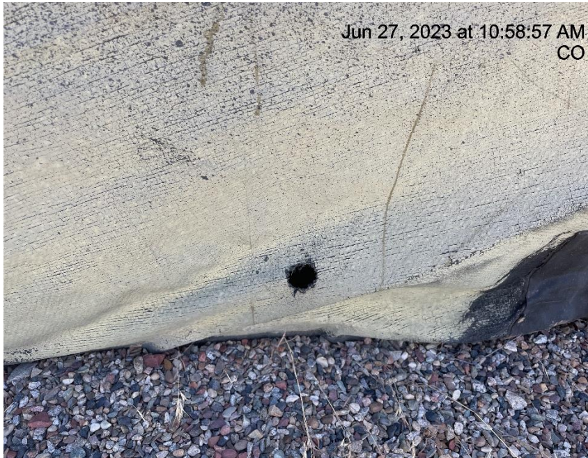
Photo # 2067 Hole in liner/liner needs maintenance
