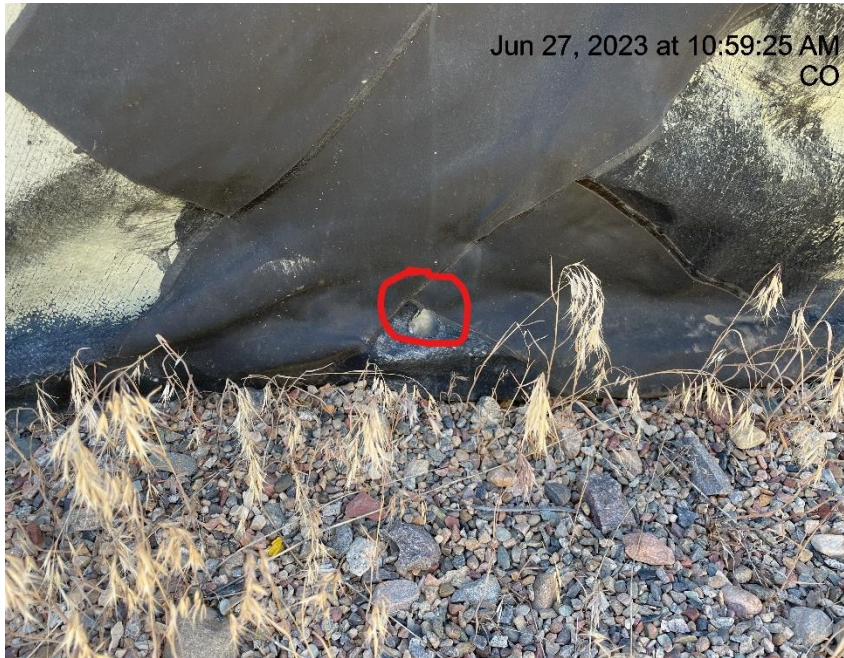
Photo # 2069 Hole in liner/liner needs maintenance
