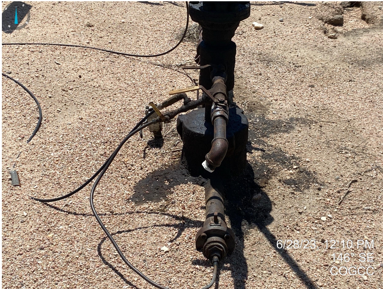
Photo 10. Stained soil at wellhead requires proper cleanup and disposal .
