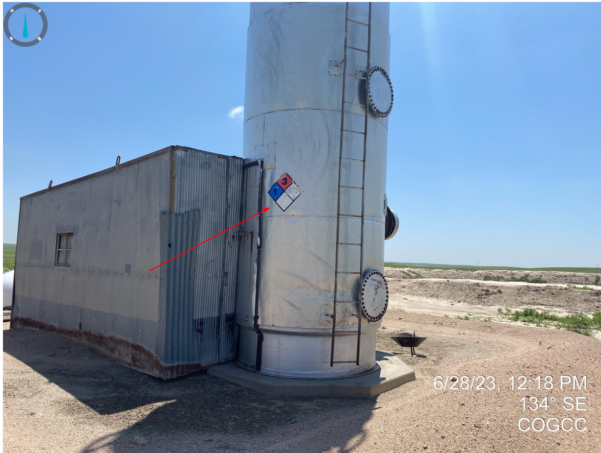
Photo 9. NFPA placard not legible and requires replacement.
