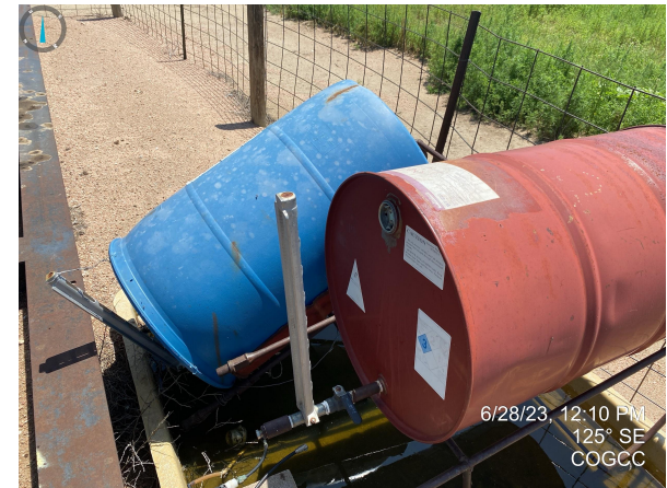
Photo 3. No wildlife protection equipment observed around secondary containment and tank labels are peeling, faded, cracked and/or not legible.
